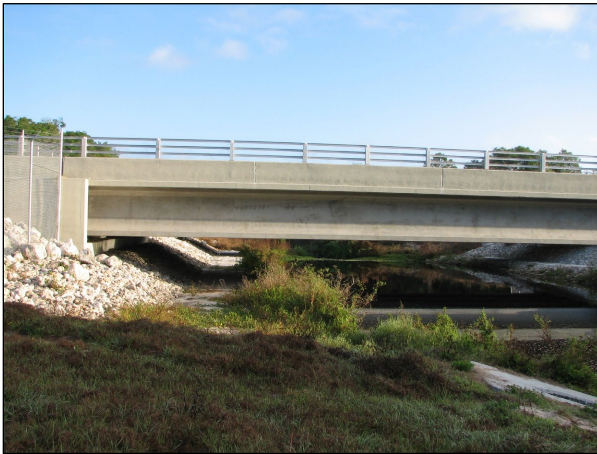
Figure 17 – 1 Bridge with Shelves for Wildlife
