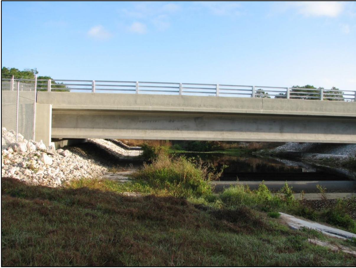
Figure 17 – 1 Bridge with Shelves for Wildlife
