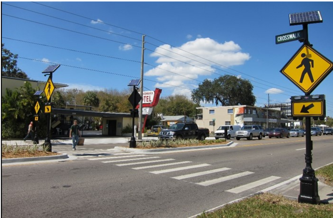
Figure 8 – 8 Pedestrian Median Refuge with Rectangular Rapid Flashing Beacons (RRFB)
