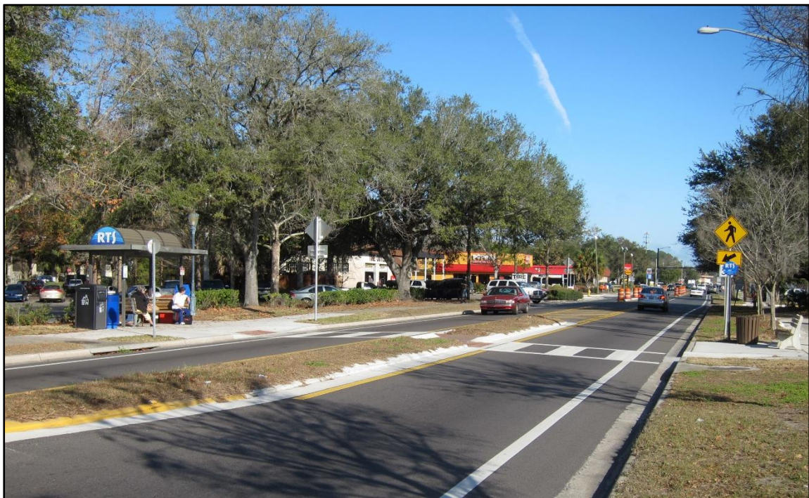
North Main Street, Gainesville, FL
