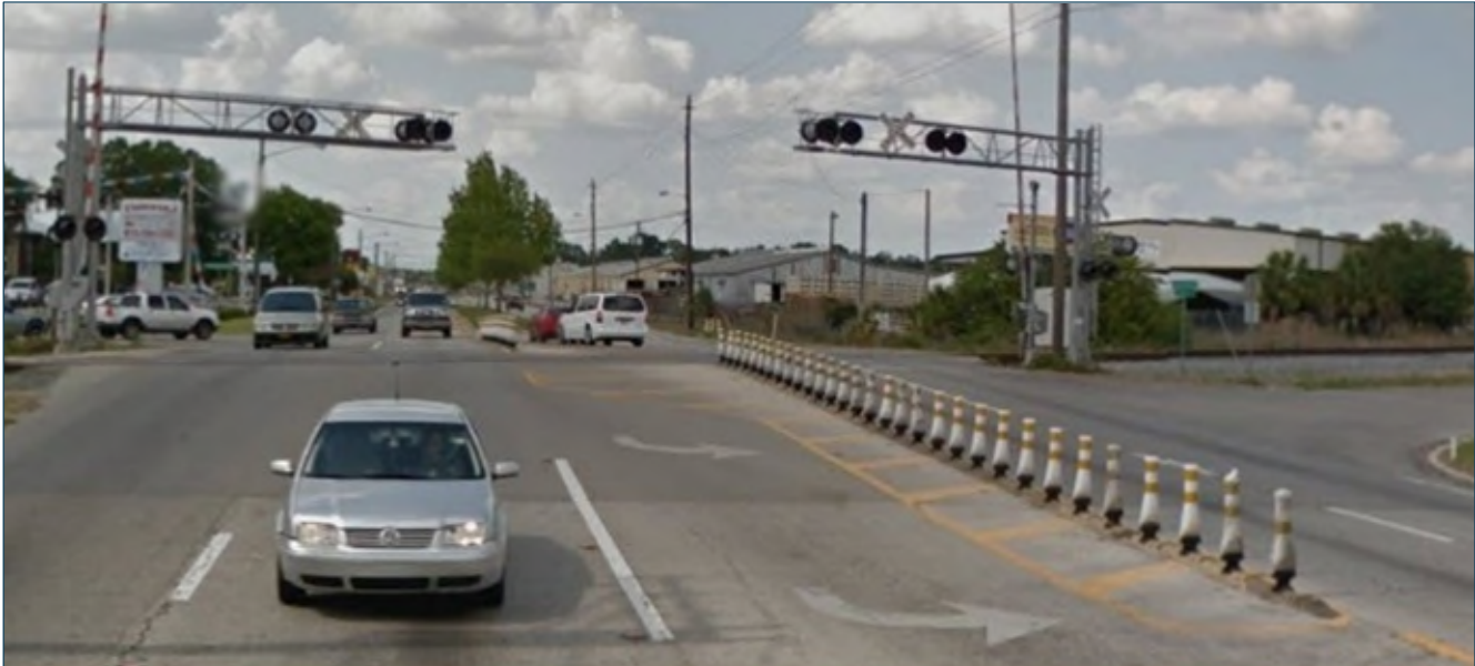
Figure 7-2 Flush Median Channelization Devices
