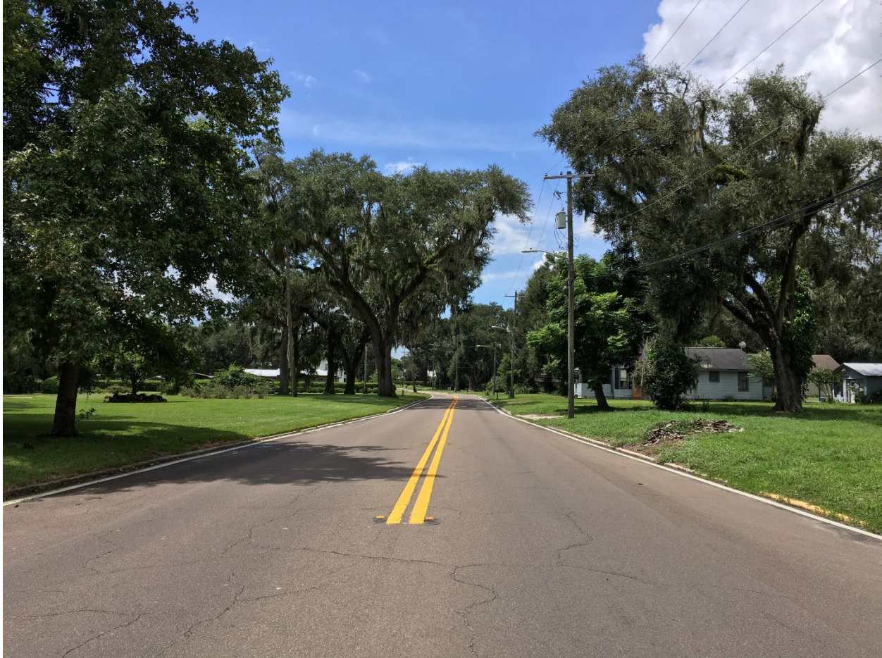
Photo by FDOT District 1
