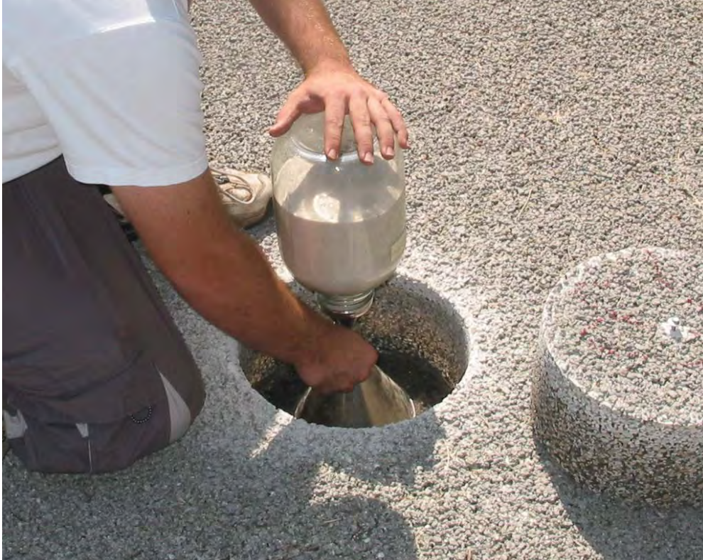
Figure 10: Performing Sand Cone Test
