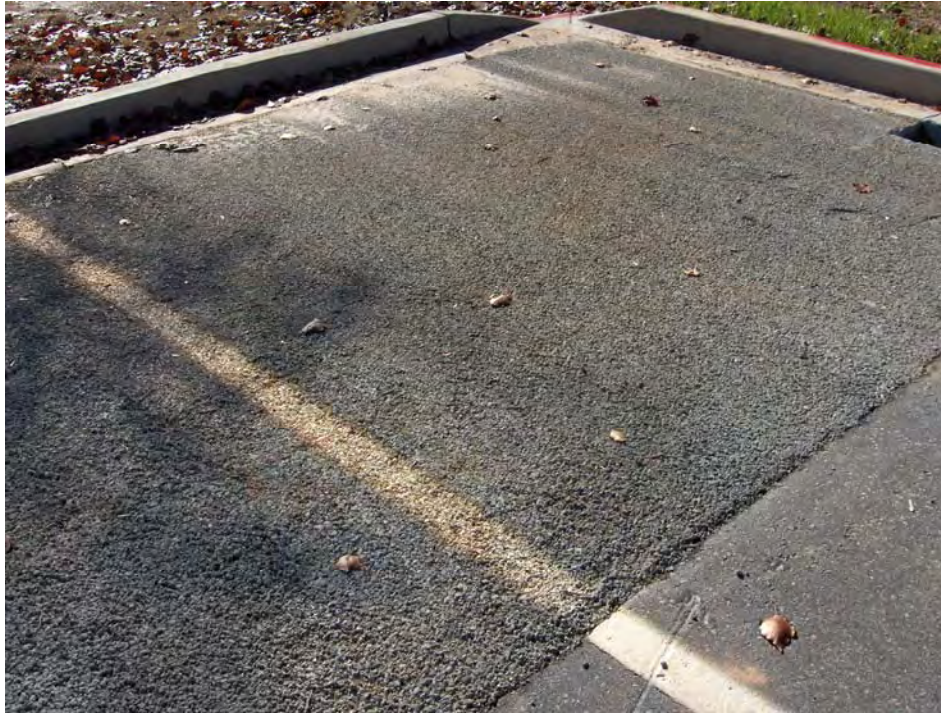
Figure 31: Cleveland Park Parking Lot Pavement
