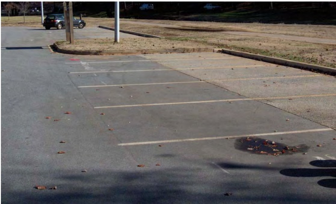
Figure 30: Cleveland Park Parking Lot
