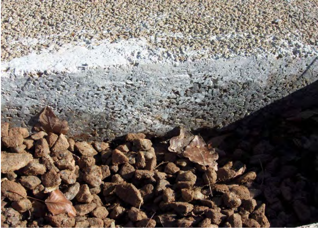
Figure 32: Cleveland Park Parking Lot Reservoir
