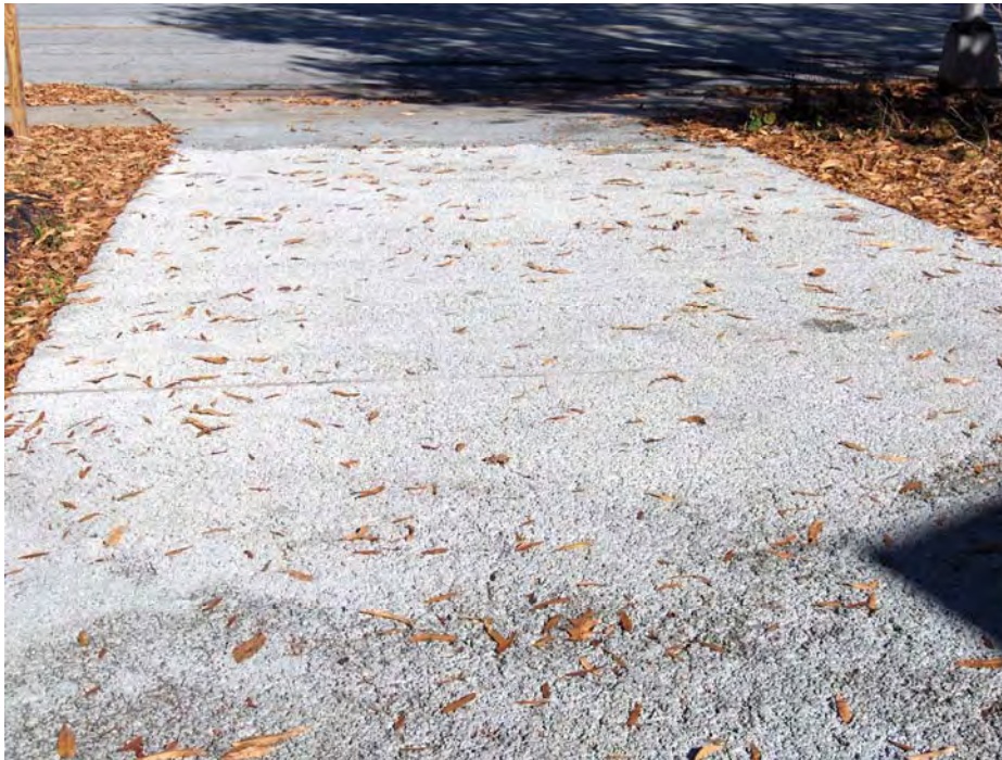
Figure 26: Southface Institute Parking Lot
