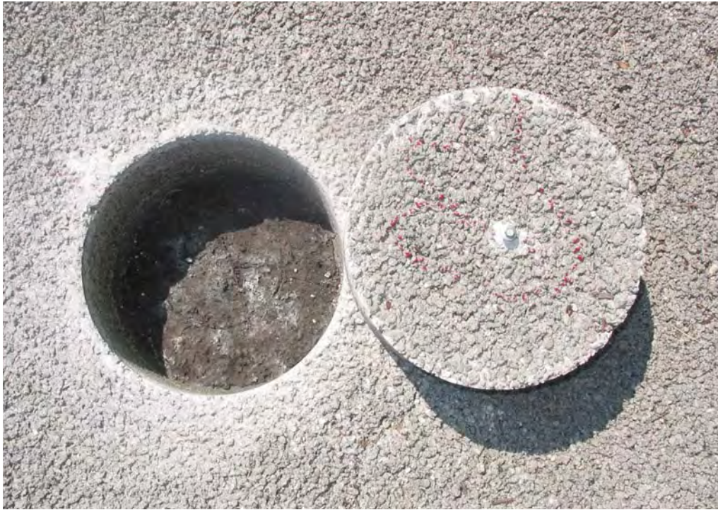
Figure 8: Pervious Concrete Pavement Core
