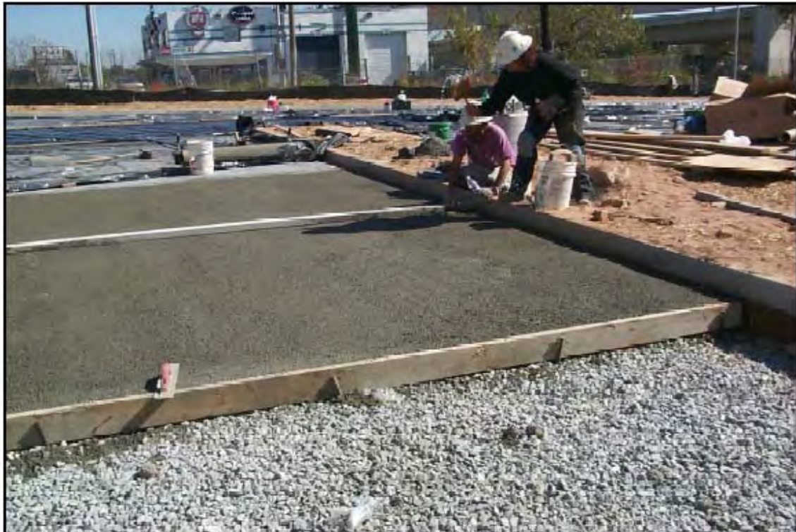
Figure 2: Typical Porous Concrete Installation
