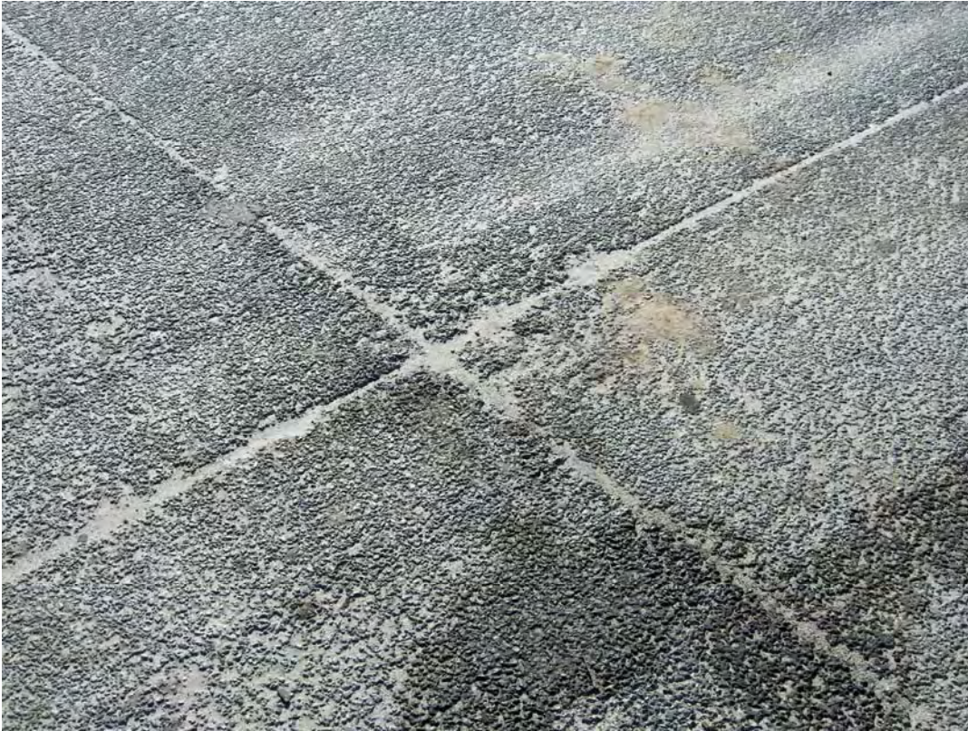
Figure 35: Effingham County Landfill Pervious Pavement
