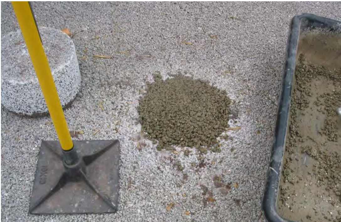
Figure 11: Repair of Concrete Core Area
