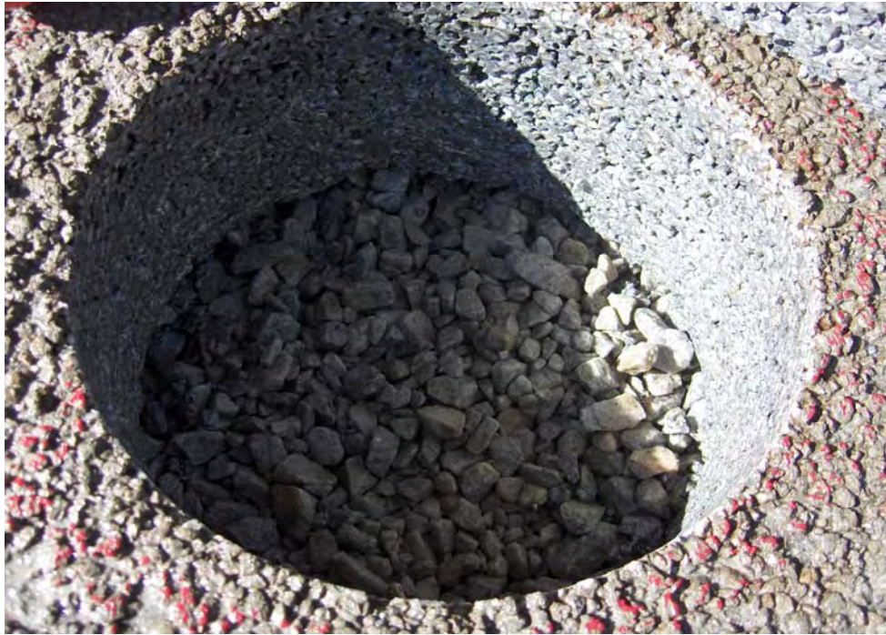
Figure 27: Southface Institute Gravel Subbase
