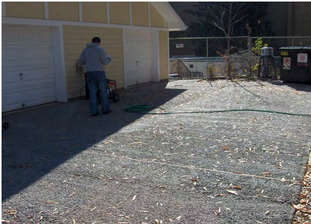
Figure 28: Southface Institute Parking Lot
