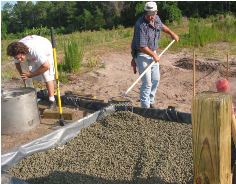
Figure 3: Stormwater Academy Porous Concrete Test Cell Installation
