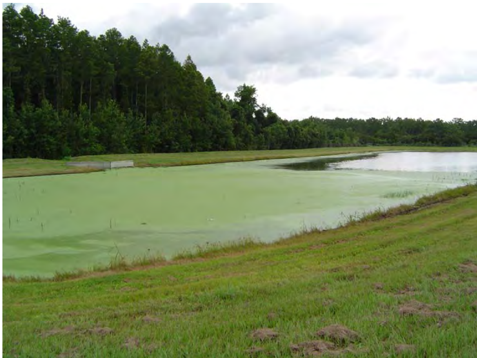
S.R. 417-4 Pond: View from northwest corner facing southeast.
