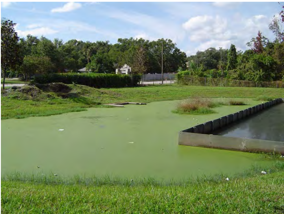
Horatio Avenue and Via Tuscany No. 2: View from southeast corner.
