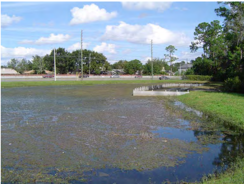
University Blvd and Hall Road Pond: View from southwest corner.
