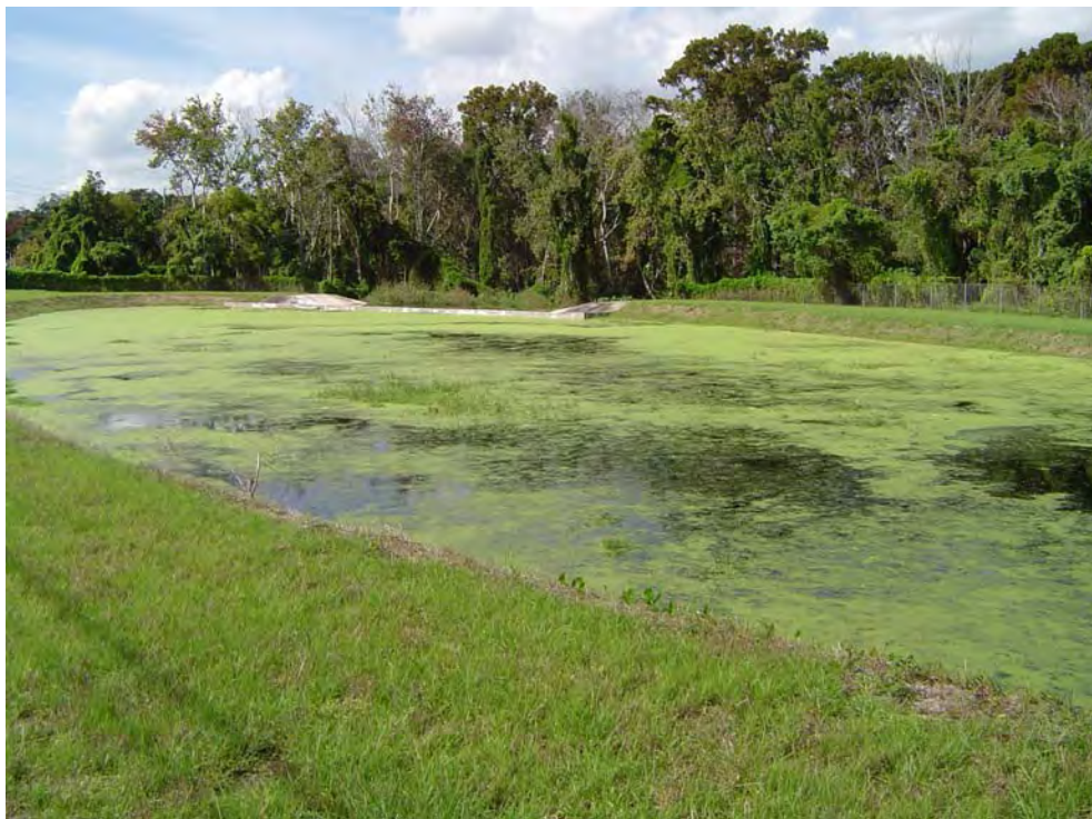
Horatio Avenue and Via Tuscany No. 1: View from southeast corner.
