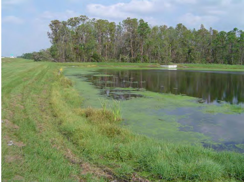
S.R. 417-5 Pond: View from southwest corner.
