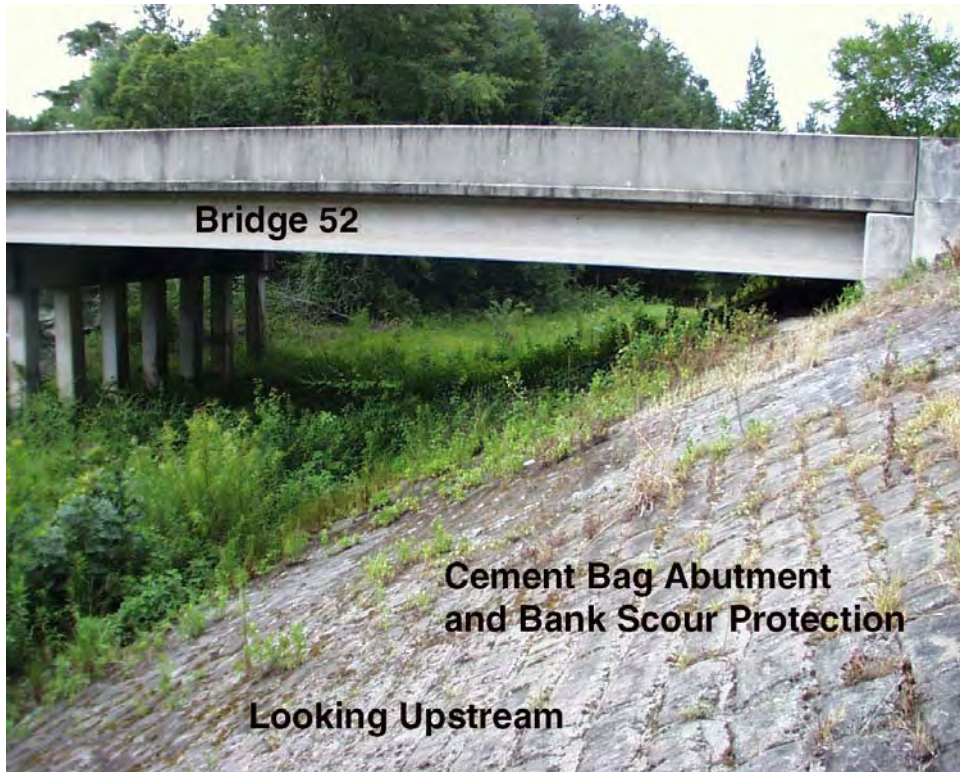
Figure C 1. Bridge 52 East Abutment
