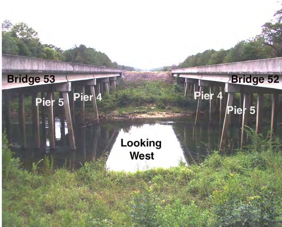
Figure 6. Bridges 52 and 53 Looking West
