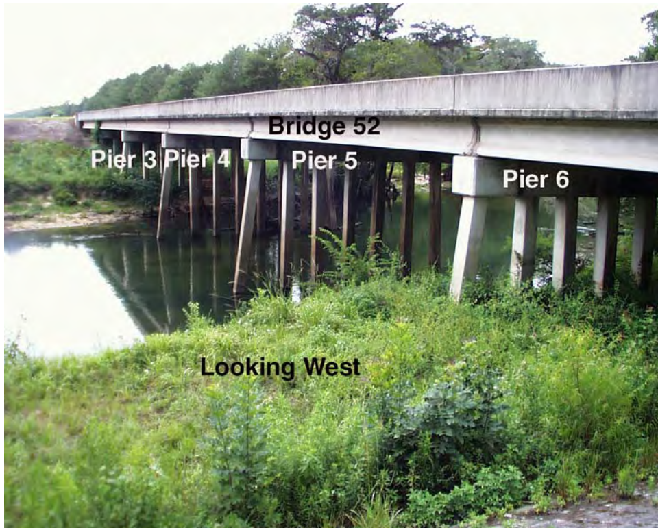
Figure C 2. Bridge 52 Looking West 3.
