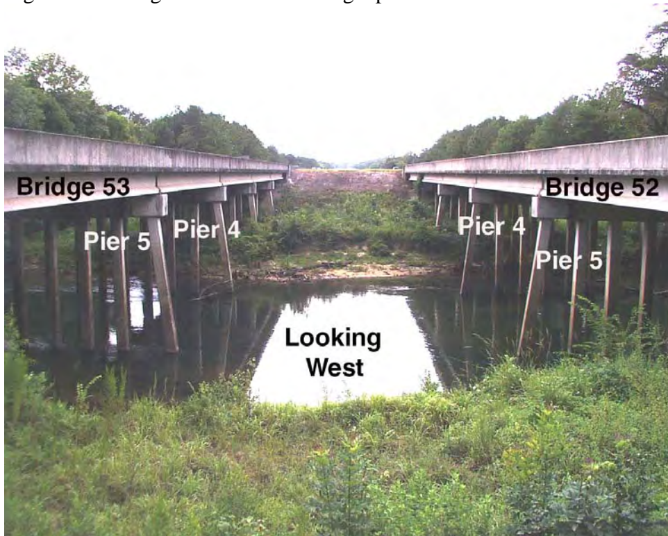
Figure C 10. Bridges 52 and 53 Looking West.
