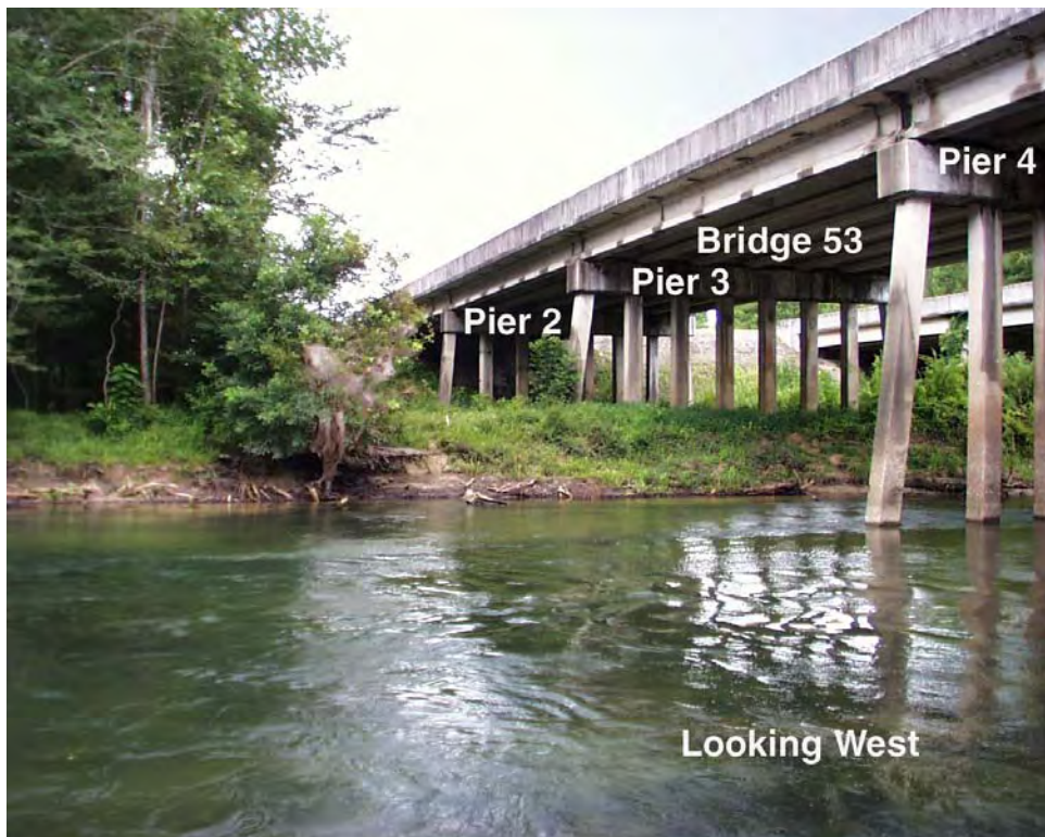
Figure C 6. Bridge 53 Looking West.
