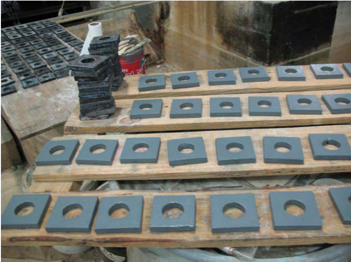
Figure 37. Spacers primed and painted.
