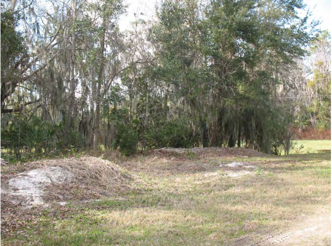
Figure 39 Trees removed for crane maneuvering space.
