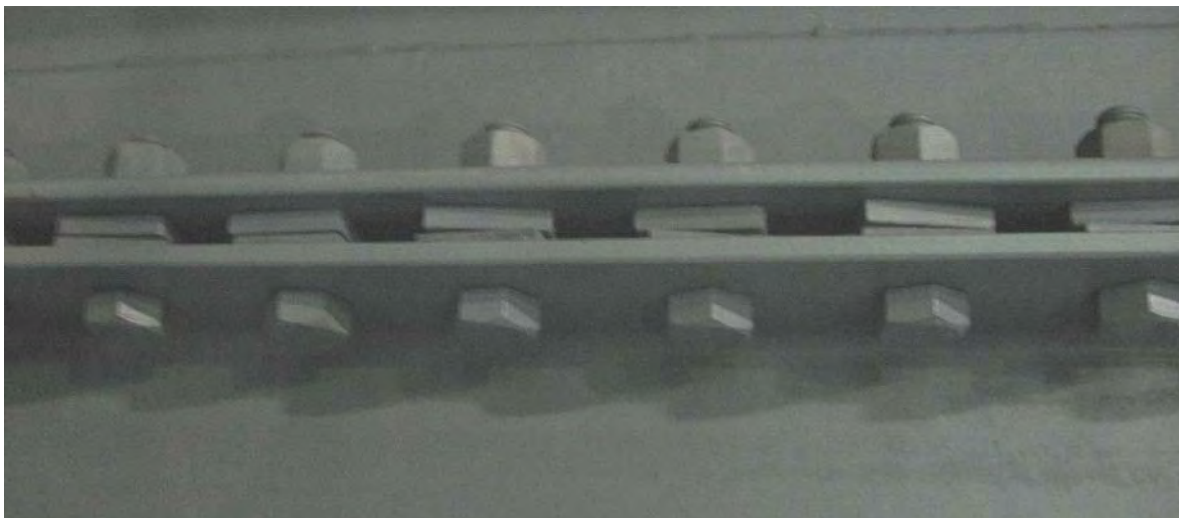
f) Close up of fastened nuts and bolts
