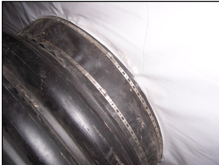
Figure 9: Installed rubber membrane sealing system.
