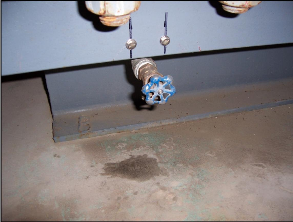
Figure 23: French drain release valve.
