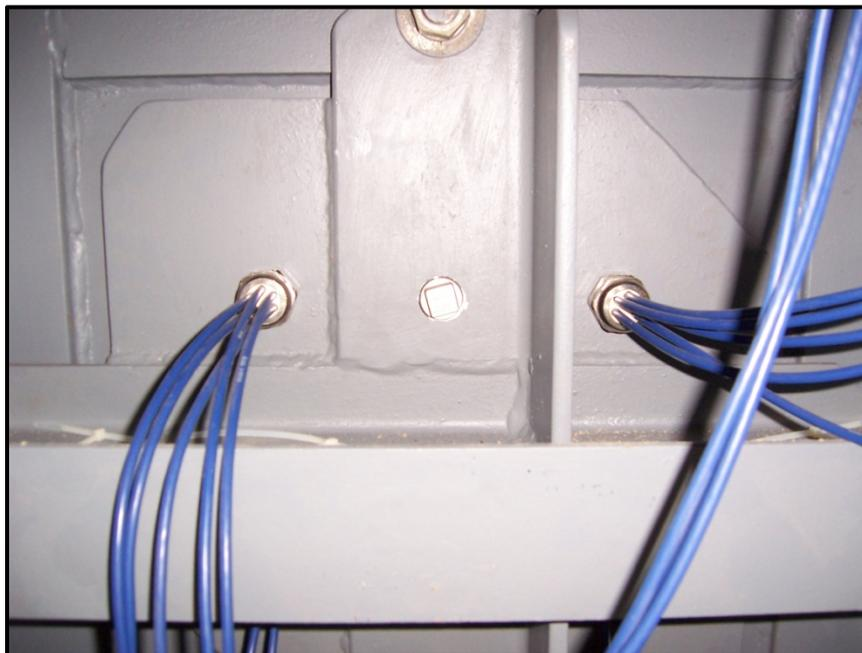
Figure 6: Completed routing of instrumentation wiring (view from outside).
