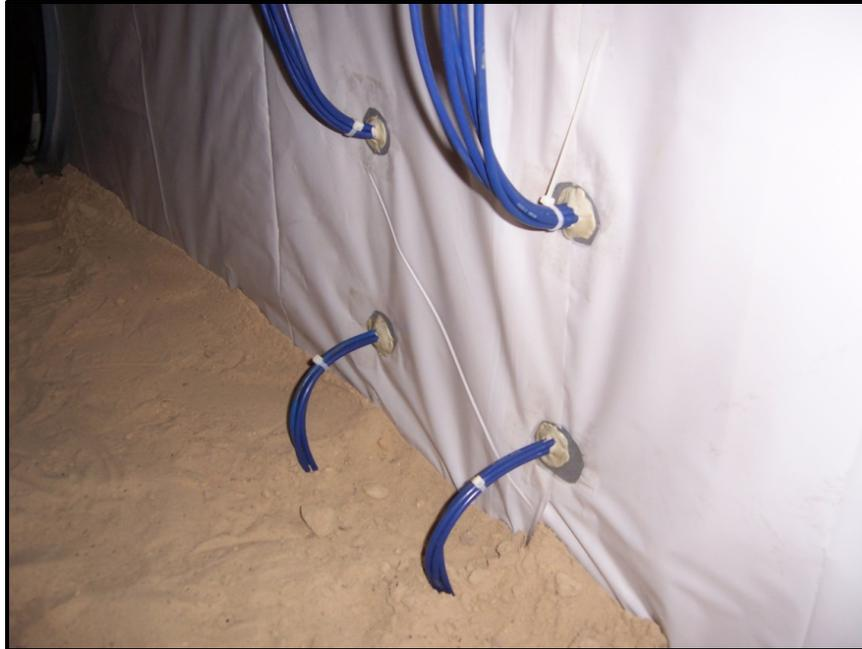
Figure 5: Completed routing of instrumentation wiring with sealant (view from inside).
