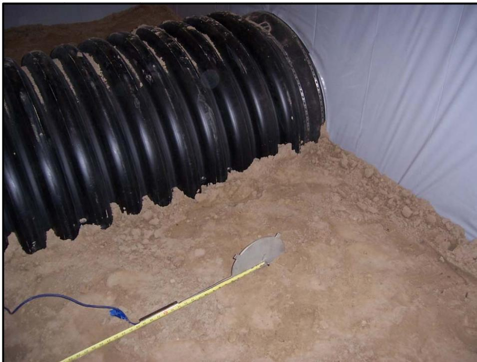
Figure 13: Placement of SS2 pressure cell.
