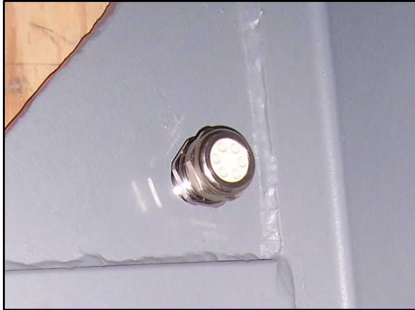
Figure 5: Instrumentation wiring guide.
