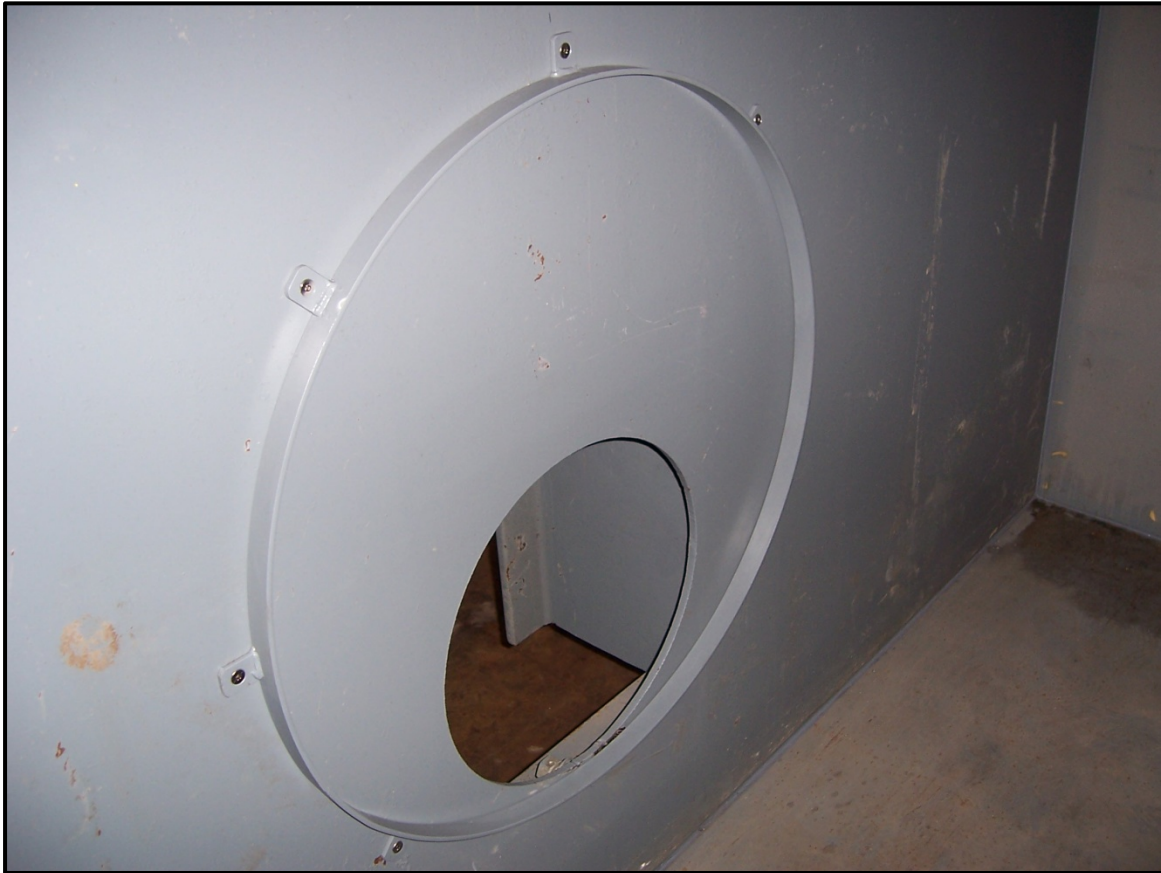
Figure 3: Completed wall flange for sealing system.
