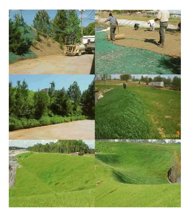
Figure AIII-7: Polymer-enhanced Turf Reinforced Matting.
