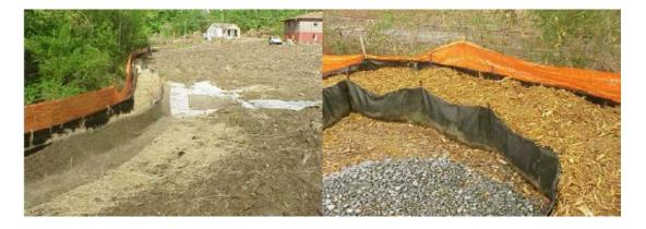
*Limitations*: Inflow values must not exceed outflow values. Suggested outflow value is to be greater than 70 *gpm/sq. ft* of silt fence areas. This implies that the standard woven or needle punched silt fence materials may not be adequate. A monofilament woven material may suffice for low flows.
