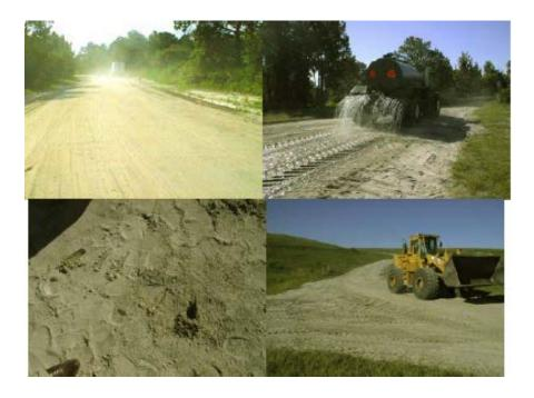
Figure AIII-29: Polymer-enhanced Dust Suppression.
