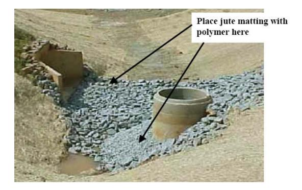
*Limitations*: It will only work well when the rock anchors the matting. Unless is maintained, the treated water flow through the jute matting may cause blockage of the rock barrier around the riser pipe.
