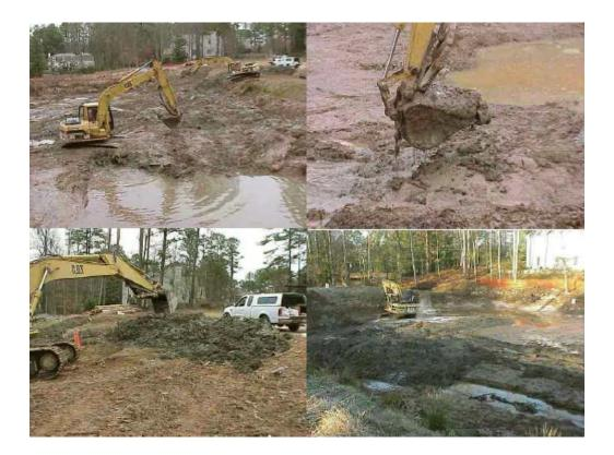
Figure AIII-28: Polymer-enhanced Mud and Sediment Removal.
