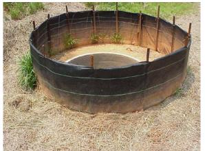
Figure AIII-12: Polymer-enhanced erosion control around drop inlet.
