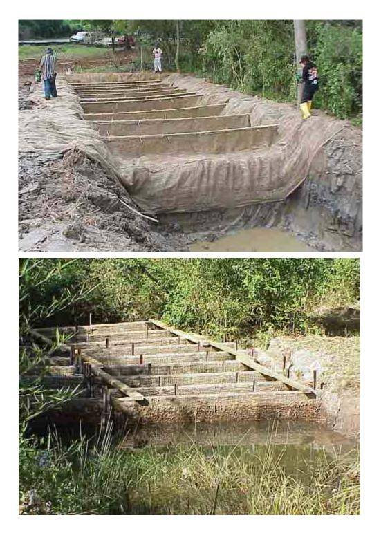
*Limitations*: It is to be noted that this application is for "polishing up" the water after it has undergone maximum treatment to remove sediment. This application is not adequate water clarity control by itself, it is intended to be used in conjunction with other stormwater treatment systems.
