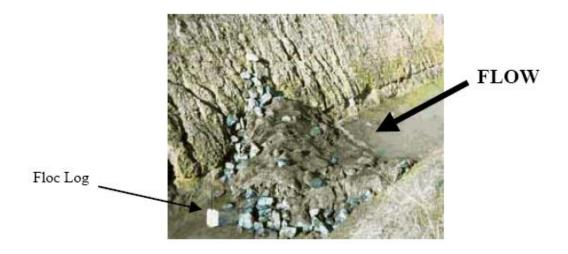
Figure AIII-16: Polymer-enhanced Check Dams.
