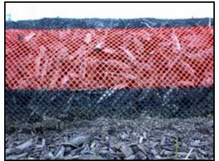
Detail of compost-filled mesh sock (Source: Filtrexx, 2006)
