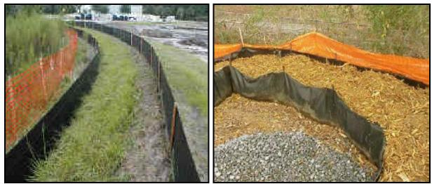
SRB prior to placement of mulch barrier (Source: Florida Dept. of Envr. Protection, 1988) SRB with shredded wood mulch and polymer (Source: Manoj Chopra, 2006)
