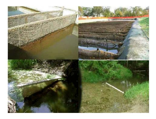
Figure AIII-25: Polymer-enhanced Particle Curtains.
