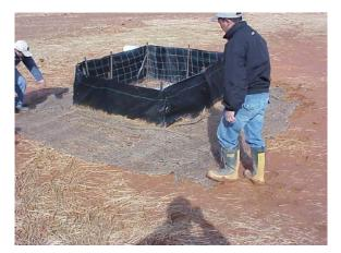
*Limitations*: Inflow values must not exceed outflow values. Suggested outflow value is to be greater than 70 gpm/sq. ft of silt fence areas. This implies that the standard woven or needle punched silt fence materials may not be adequate. A monofilament woven material may suffice for low flows. In addition, proper installation is critical.
