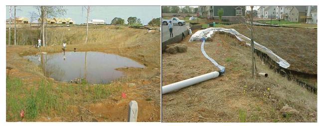
Figure AIII-2: The water was pumped out of the sediment pond.
