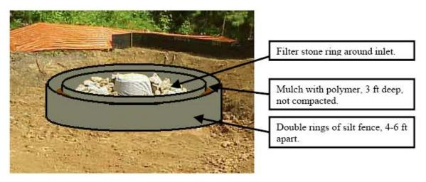
*Limitations*: Inflow values must not exceed outflow values. Suggested outflow value is to be greater than 70 *gpm/sq. ft* of silt fence areas. This implies that the standard woven or needle punched silt fence materials may not be adequate. A monofilament woven material may suffice for low flows.
