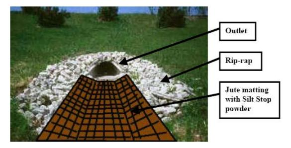
*Limitations*: If riprap is being placed under the jute, there may be damage to the material for significant flows. It is for this reason that assessing the shear stress and velocity needs to be completed as does placing rock anchors on top of the material.
