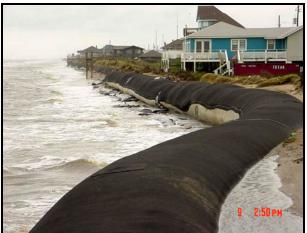
Sandsock, sand-filled tubular geotextile (Source: Surfrider Foundation, 2006)
