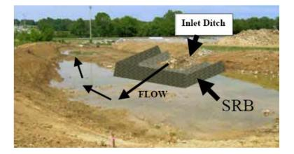
*Limitations*: Inflow values must not exceed outflow values. Suggested outflow value is to be greater than 70 *gpm/sq. ft* of silt fence areas. This implies that the standard woven or needle punched silt fence materials may not be adequate. A monofilament woven material may suffice for low flows.
