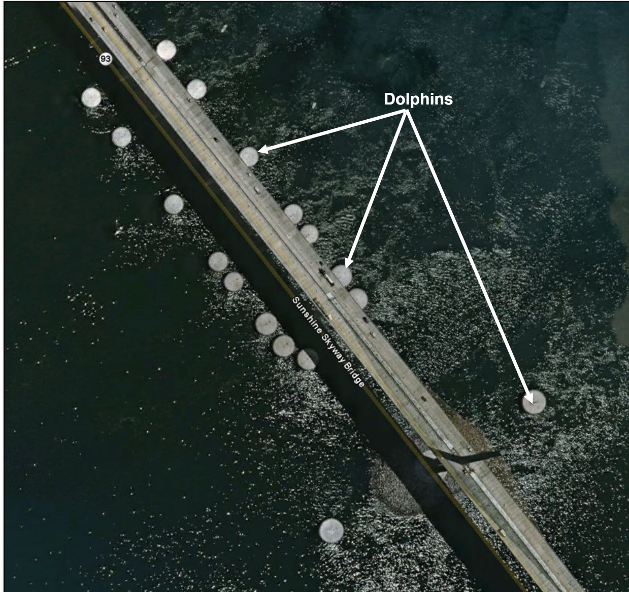
Figure 5.1-10: Dolphin Pier Protection at the Sunshine Skyway Bridge
