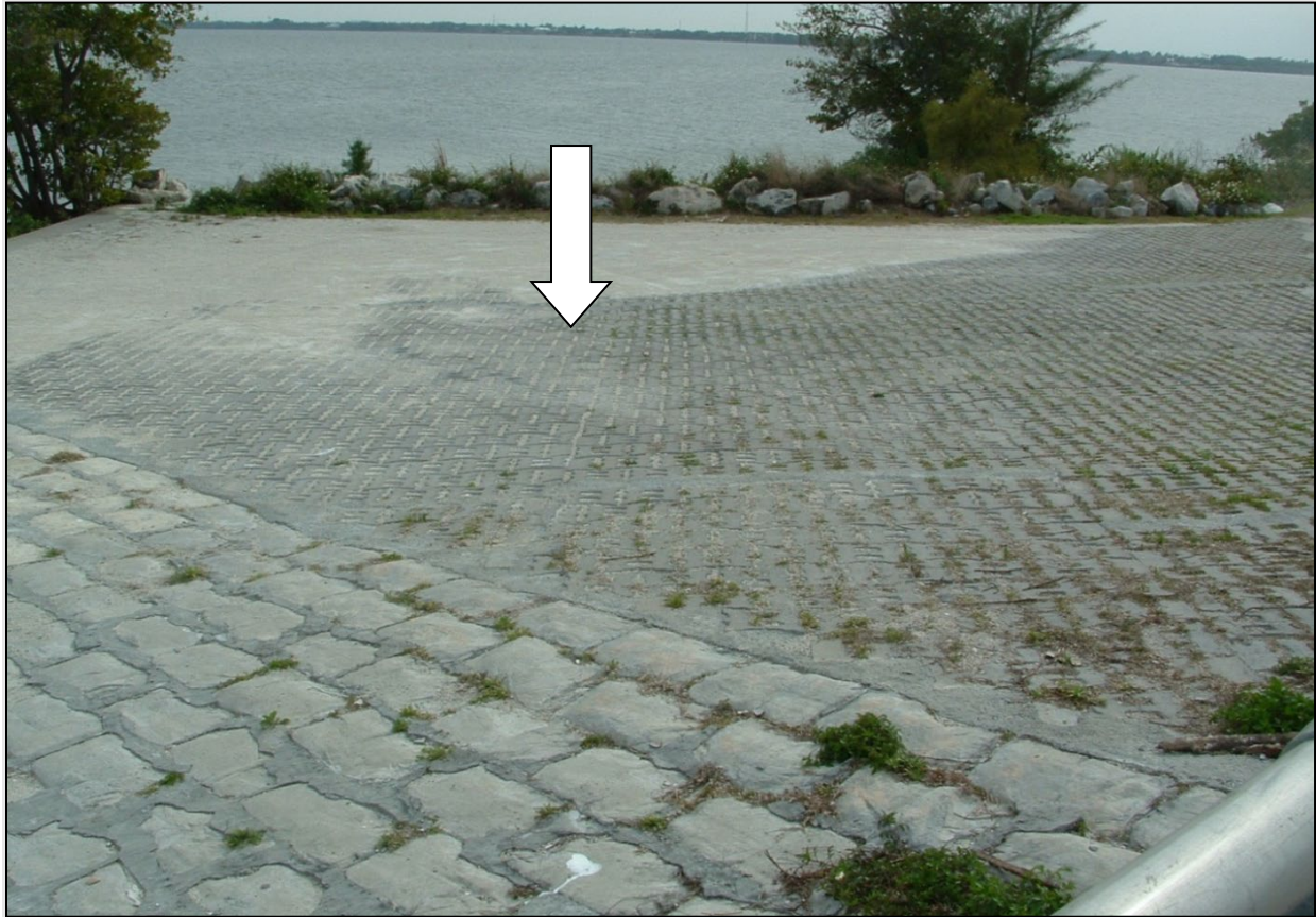
Figure 5.5-14: Example of Articulating Concrete Block Abutment Protection
