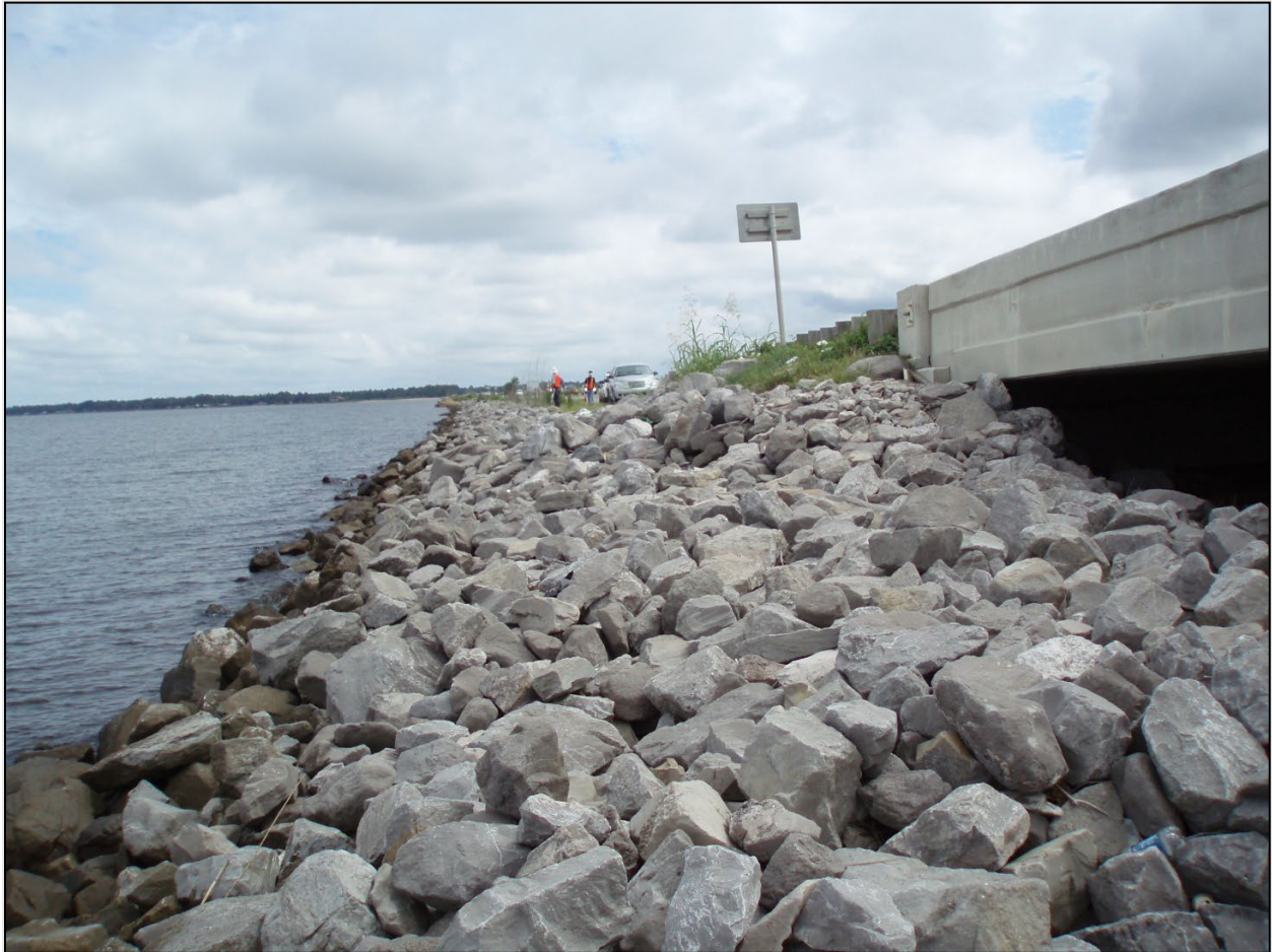
Figure 5.5-13: Example of Rubble Riprap Abutment Protection
