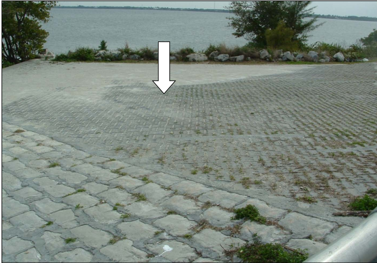
Figure 5.5-14: Example of Articulating Concrete Block Abutment Protection
