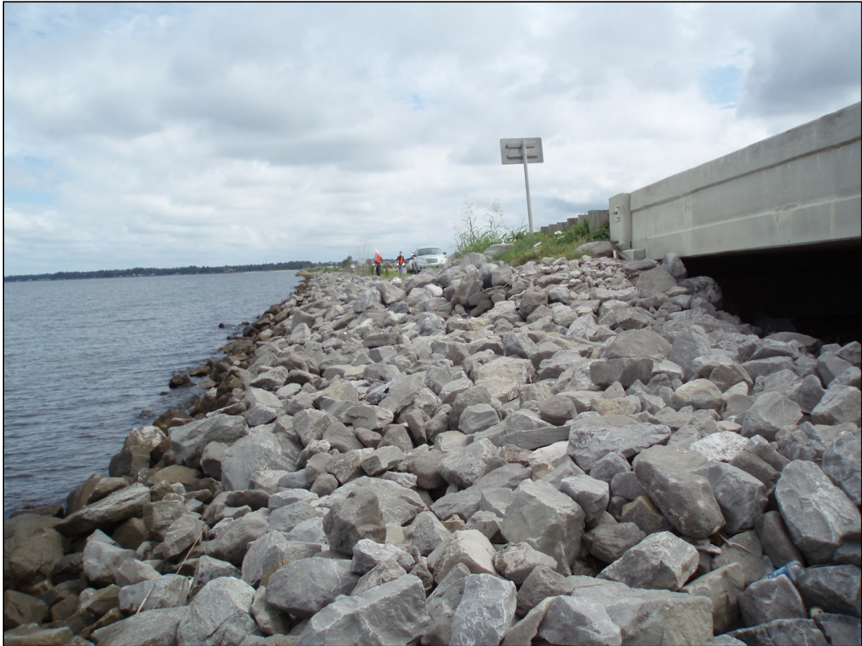
Figure 5.5-13: Example of Rubble Riprap Abutment Protection
