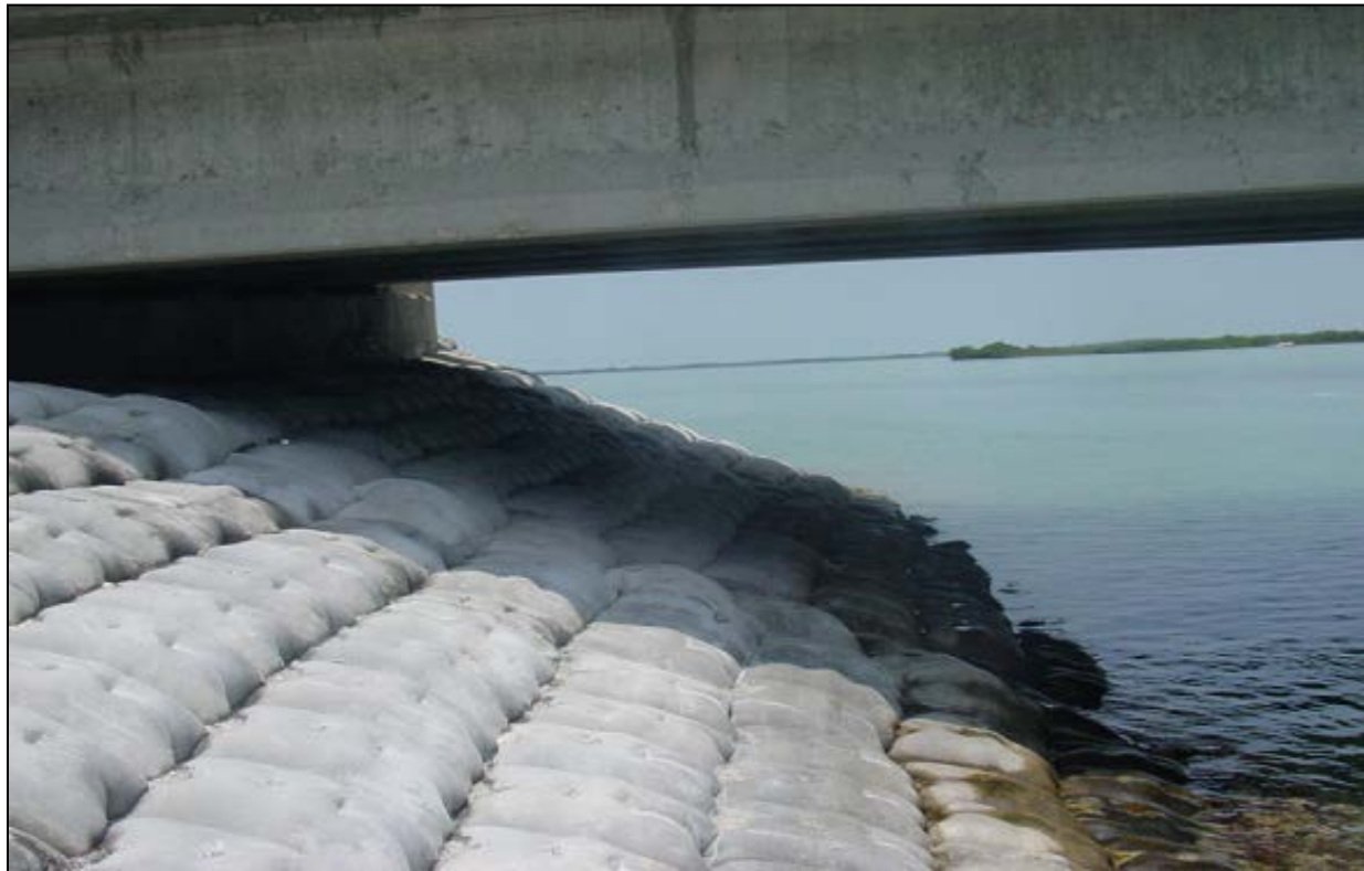
Figure 5.5-15: Example of Fabric Formed Revetment Abutment Protection
