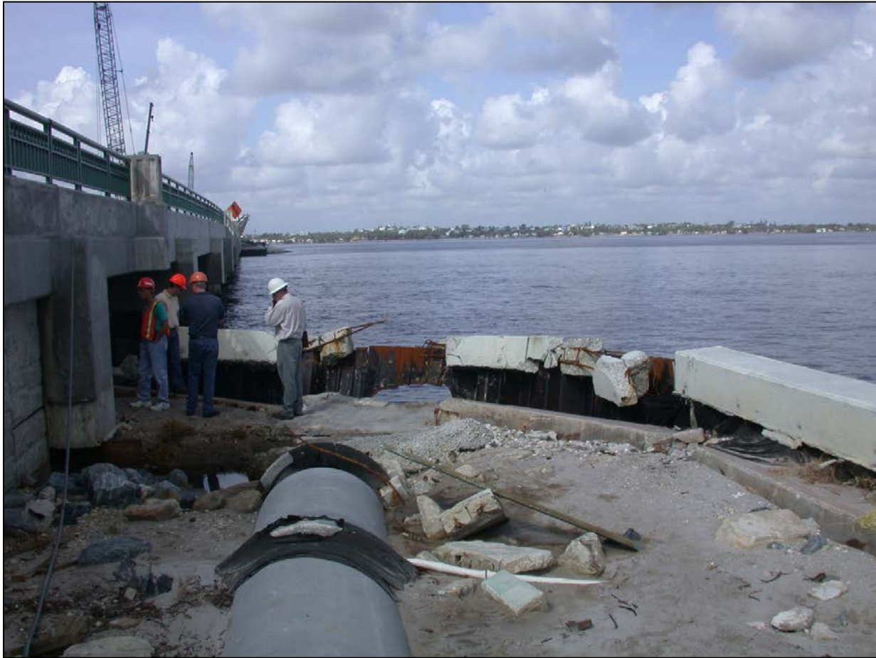
Figure 5.5-17: Seawall Failure Following Hurricane Frances (2004)
