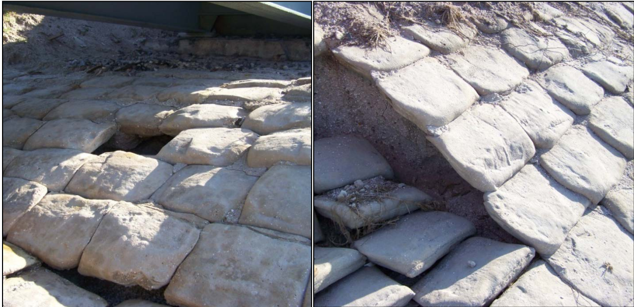
Figure 5.5-11: Damage to Sand-Cement Grouted Riprap Abutment Protection
