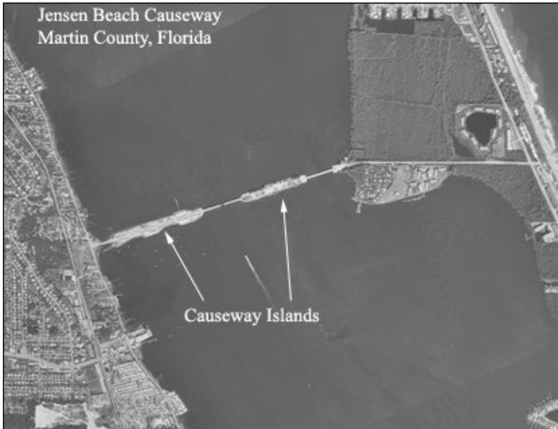
Figure 5.5-2: Example of Manmade Causeway Islands Creating a Channel Contraction
