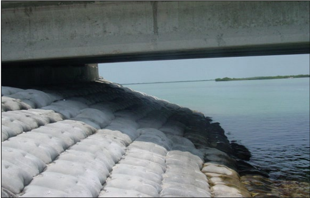
Figure 5.5-15: Example of Fabric Formed Revetment Abutment Protection
