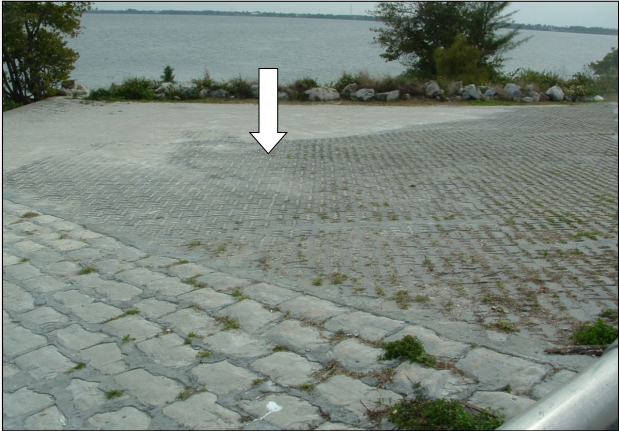
Figure 5.5-14: Example of Articulating Concrete Block Abutment Protection
