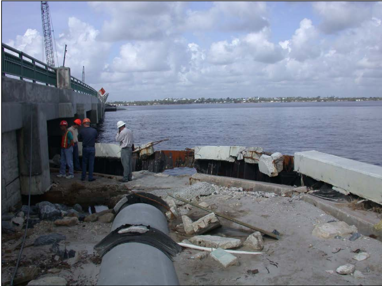
Figure 5.5-17: Seawall Failure Following Hurricane Frances (2004)
