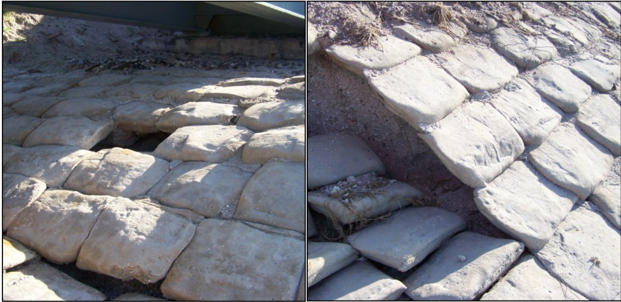
Figure 5.5-11: Damage to Sand-Cement Grouted Riprap Abutment Protection
