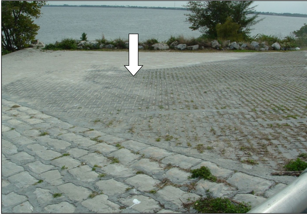
Figure 5.5-14: Example of Articulating Concrete Block Abutment Protection
