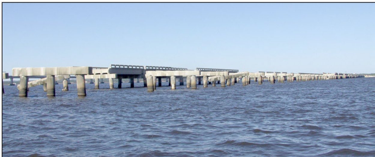
Figure 5.3-19: Damage to the I-10 Bridge over Escambia Bay during Hurricane Ivan (2004)
