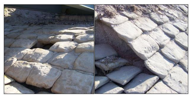
Figure 5.5-11: Damage to Sand-Cement Grouted Riprap Abutment Protection
