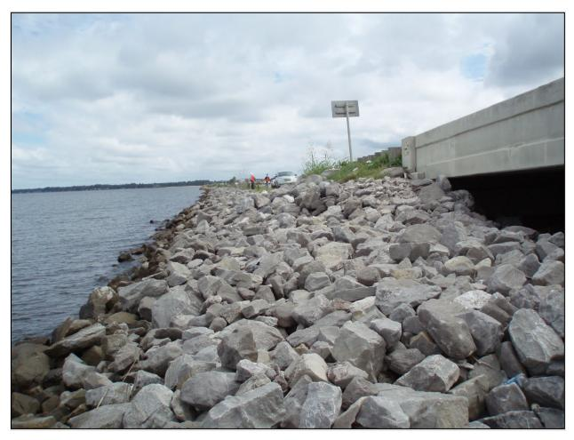
Figure 5.5-13: Example of Rubble Riprap Abutment Protection
