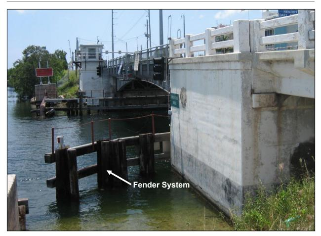
Figure 5.1-11: Fender System at the Old Jewfish Creek Bridge
