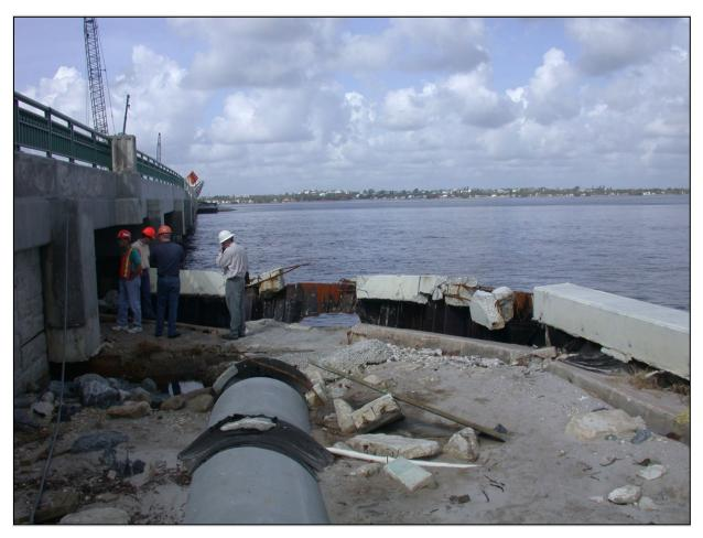
Figure 5.5-17: Seawall Failure Following Hurricane Frances (2004)
