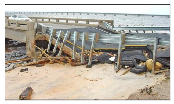
Figure 5.5-6: East Approach to the I-10 WB Bridge over Escambia Bay After Hurricane Ivan (2004)
