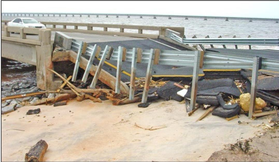
**Figure 5.5-6: East Approach to the I-10 WB Bridge over Escambia Bay After Hurricane Ivan (2004)**
