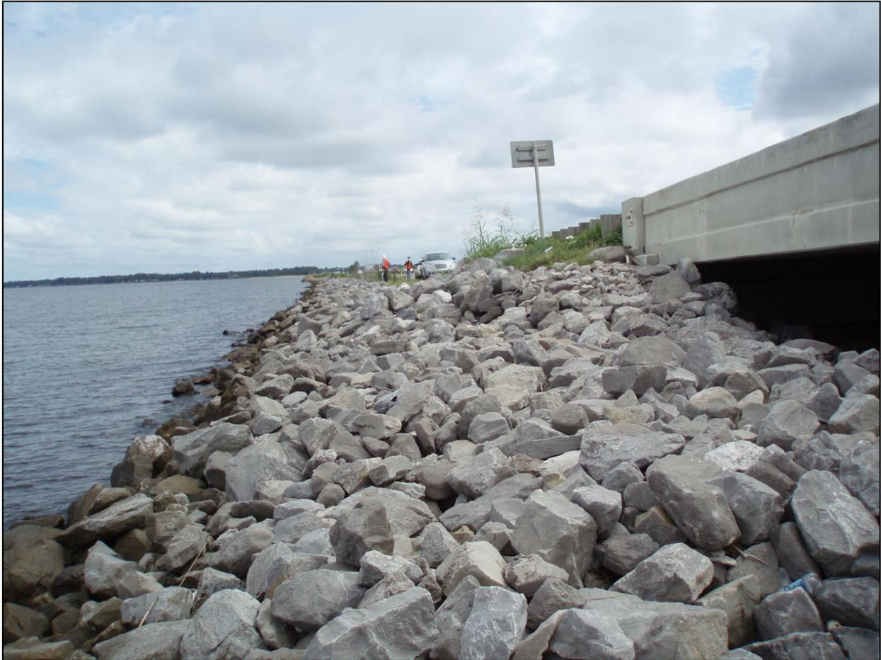
**Figure 5.5-13: Example of Rubble Riprap Abutment Protection**
