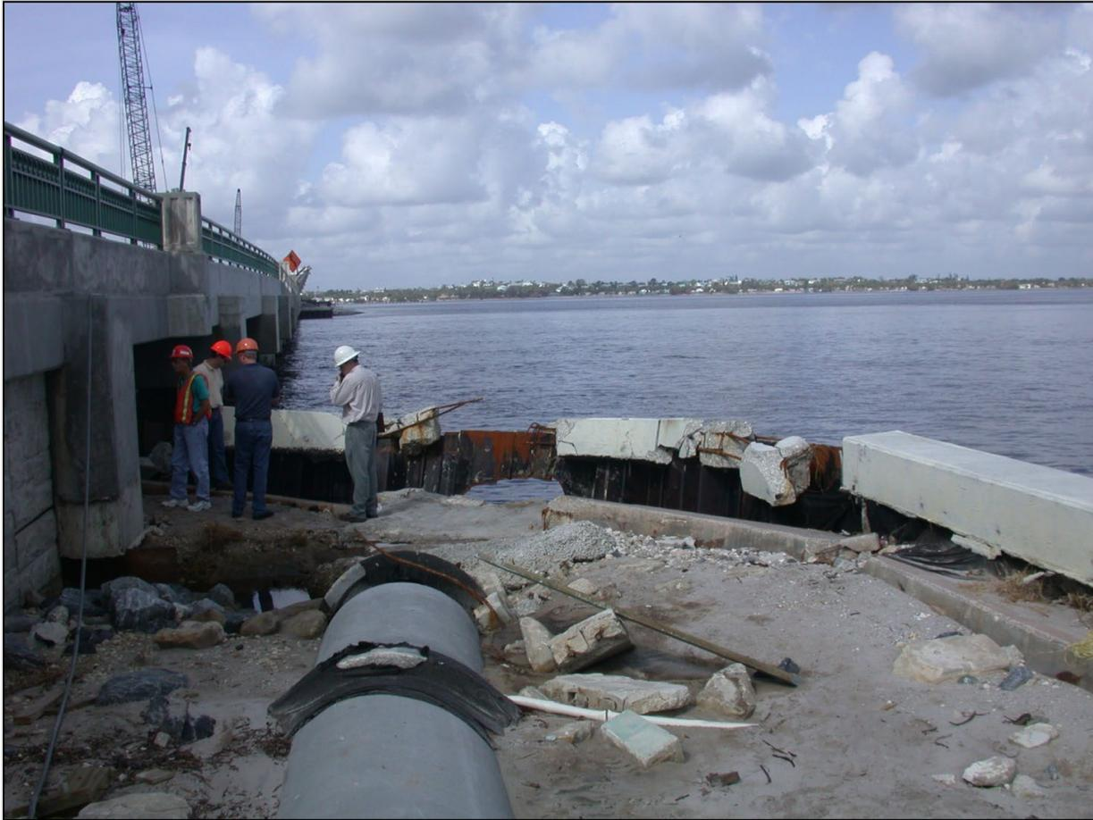
**Figure 5.5-17: Seawall Failure Following Hurricane Frances (2004)**
