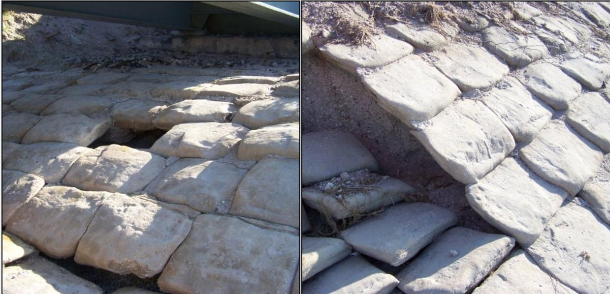
**Figure 5.5-11: Damage to Sand-Cement Grouted Riprap Abutment Protection**
