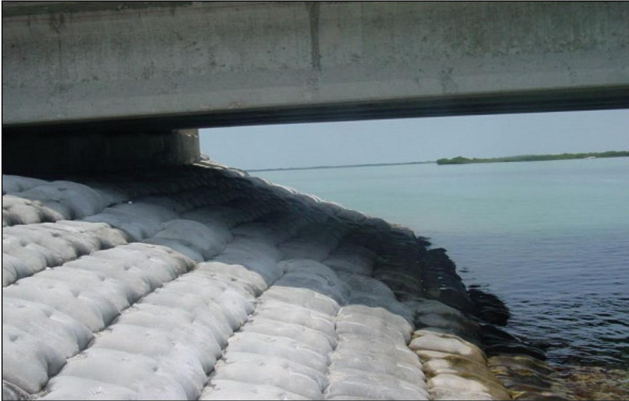
**Figure 5.5-15: Example of Fabric Formed Revetment Abutment Protection**
