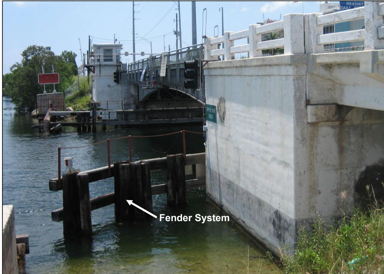
**Figure 5.1-11: Fender System at the Old Jewfish Creek Bridge**
