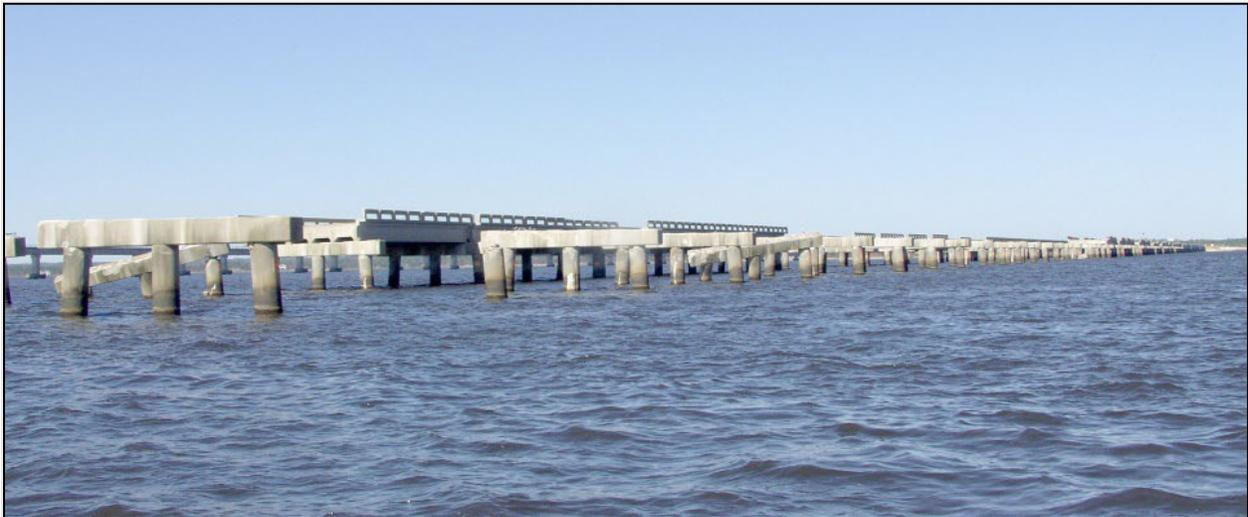
**Figure 5.3-19: Damage to the I-10 Bridge over Escambia Bay during Hurricane Ivan (2004)**
