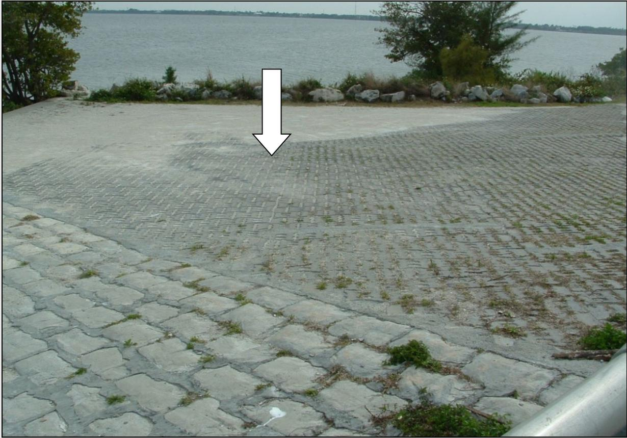
**Figure 5.5-14: Example of Articulating Concrete Block Abutment Protection**
