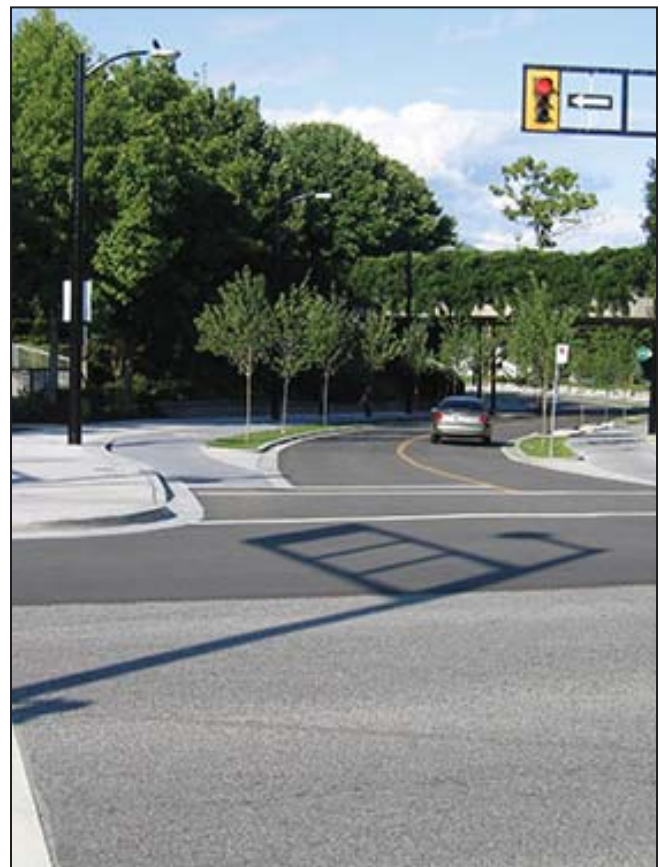
Intersections need to serve the demands of all users.
