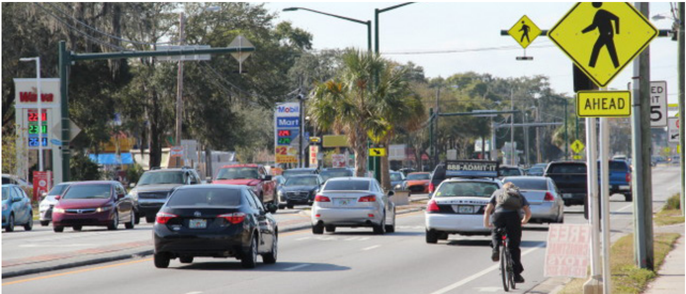
The anticipated users of a roadway and the travel patterns of those users should inform the needs and the alternatives developed for a project. Location: Fletcher Avenue, Tampa, FL Source: FDOT
