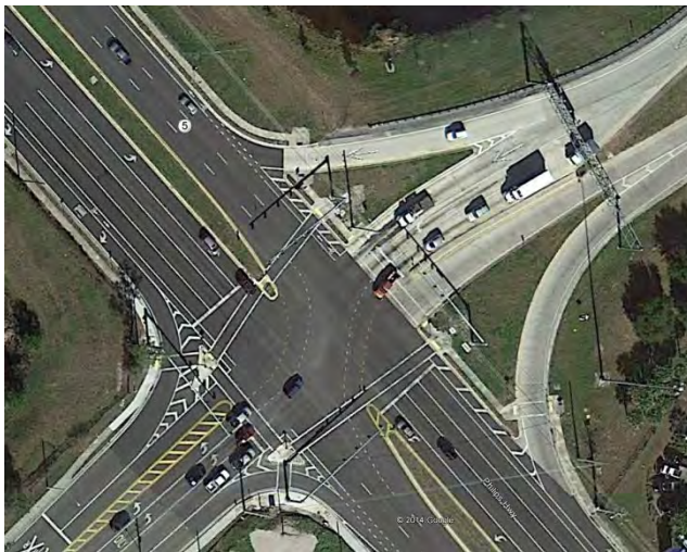
Narrow Ramp Median
