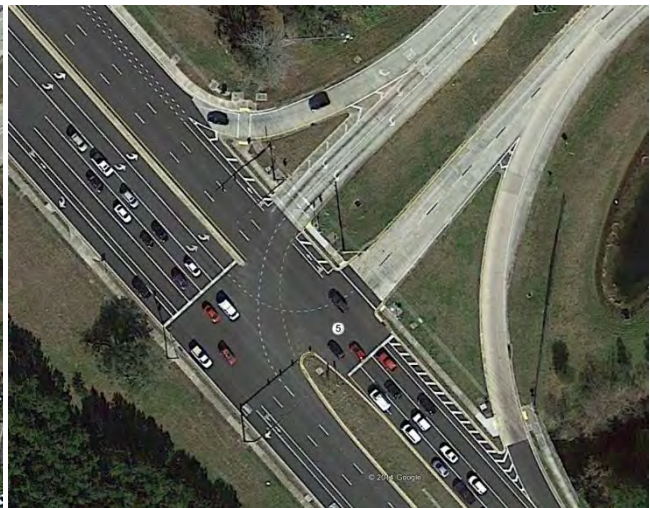
Wider Ramp Median
