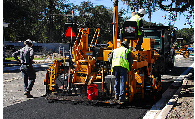
Asphalt used on roadways in Florida must meet strict specifications.
