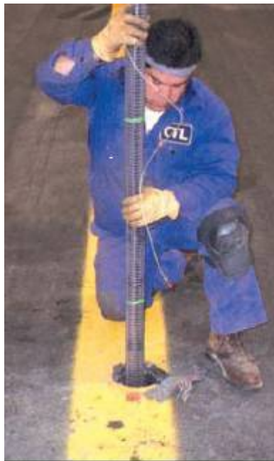
Figure 2-7. Installation of a MDD.
