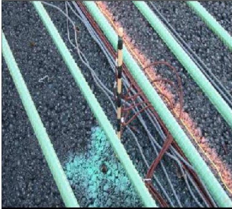
Figure 2-13. Thermocouples mounted to a “tree” awaiting PCC placement.
