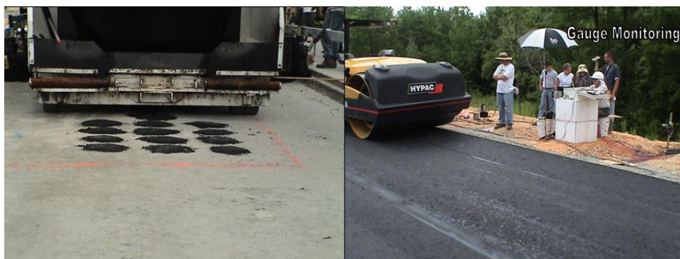
Figure 4-20. Paving over gauges.
