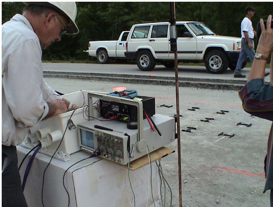
Figure 4-18. Functionality check of gauges prior to paving.
