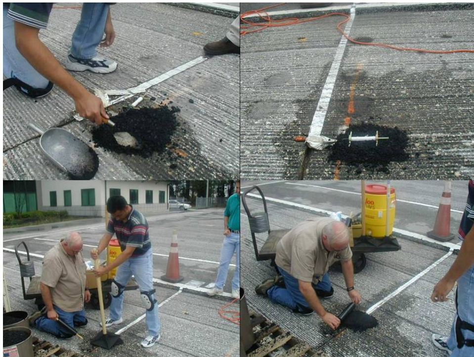
Figure 4-19. Gauge hand placement process.
