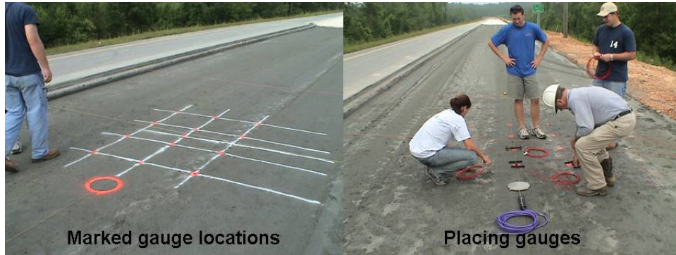
Figure 4-17. Marking and placing of gauges.
