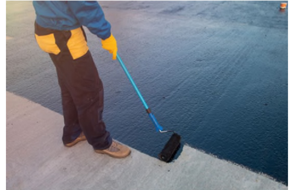
Topical waterproofing of concrete surface is mostly suitable for vertical fine cracks with a width of <math><0.005\text{ in.}/<0.127\text{ mm}</math>.
