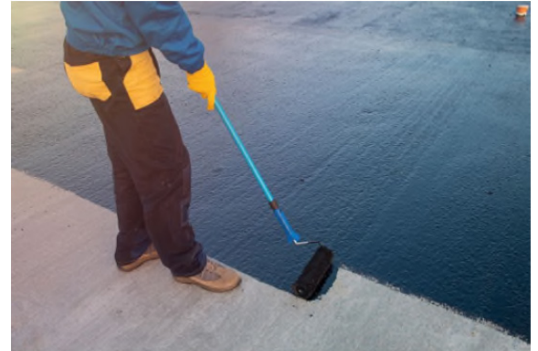
Topical waterproofing of concrete surface is mostly suitable for vertical fine cracks with a width of <math><0.005\text{ in.}/<0.127\text{ mm}</math>.
