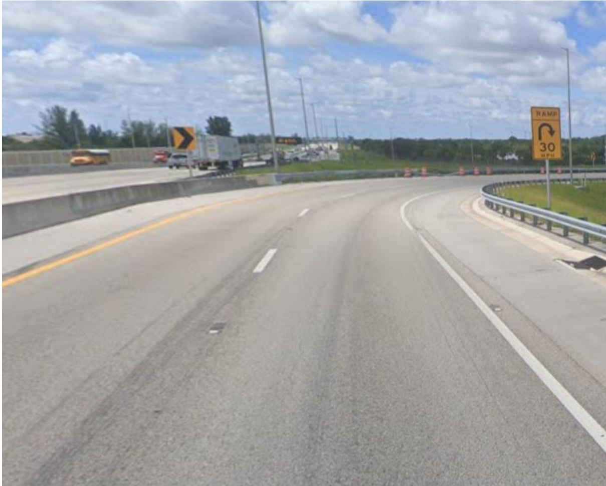
Figure 7-8: Hot-spot location 1 site image
