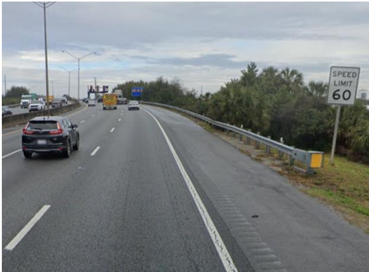
Figure 7-10: Hot-spot location 2 site image
