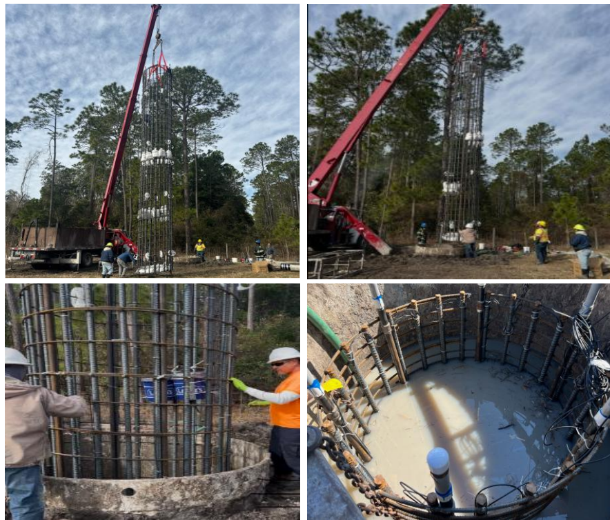
Figure 4.9 Rebar cage placement in borehole. Plastic spacers were used to maintain alignment and cover thickness of 6 inches.
