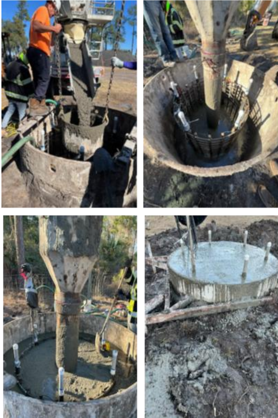
Figure 4.10 Tremie concrete casting.
