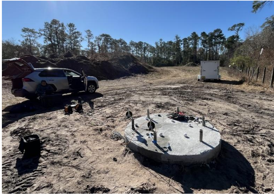
Figure 4.13 Field CSL testing setup at the Hawthorne FDOT pit showing the instrumented test shaft and on-site acquisition equipment.
