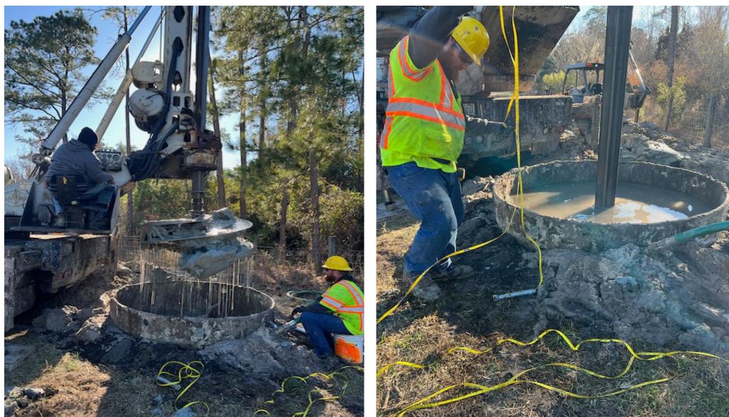
Figure 4.8 Soil drilling and slurry maintain. The completed reinforcement cage, including CSL tubes and pre-installed simulated defects, was lifted and lowered into the slurry-filled borehole using plastic spacers to maintain alignment and minimize disturbance of defect placements and tube geometry (
