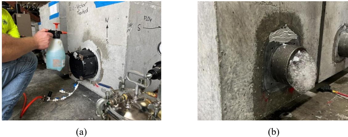
Figure 8.4. Air flow tests on S12-P-T beam: (a) Checking for leaks at the bearing plate-concrete joint at PT live end; (b) Bubbles confirming air flow at the PT dead end.
