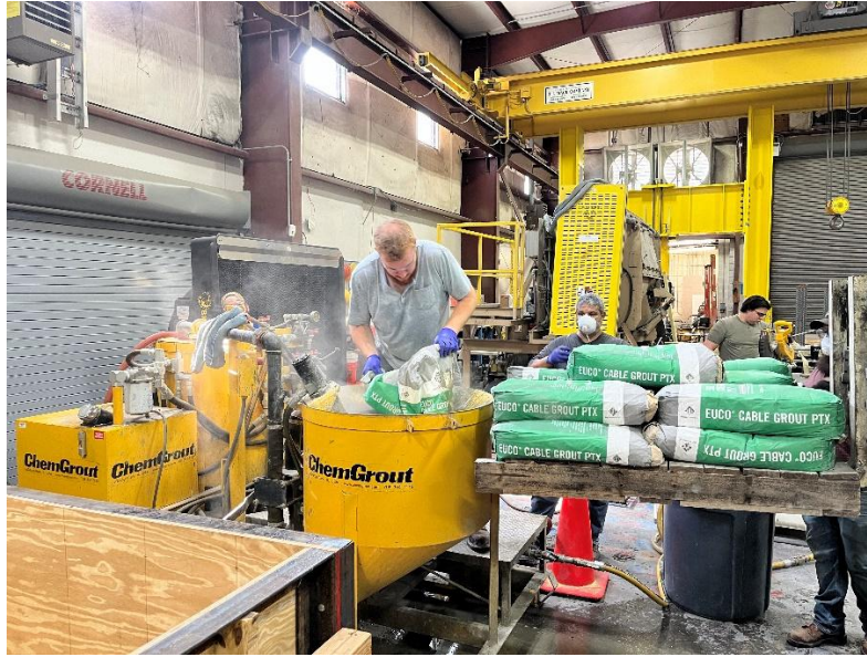
Figure 6.13. Pre-packaged grout being mixed in the colloidal grout plant.
