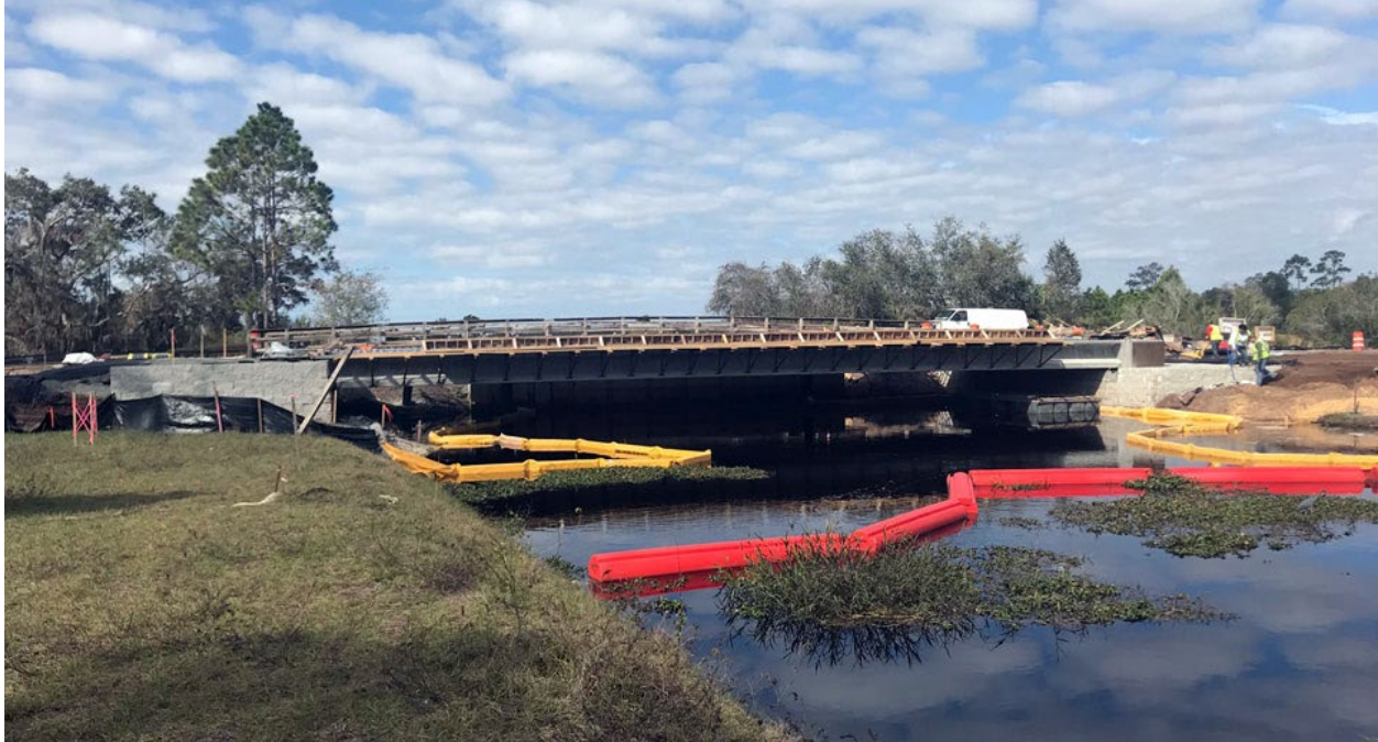
Figure 2-9. Cow Camp Bridge in Polk County, Florida. ( https://www.conteches.com/knowledge-center/case-studies/details/slug/cow-camp-road-grs-ibs-bridge ).
