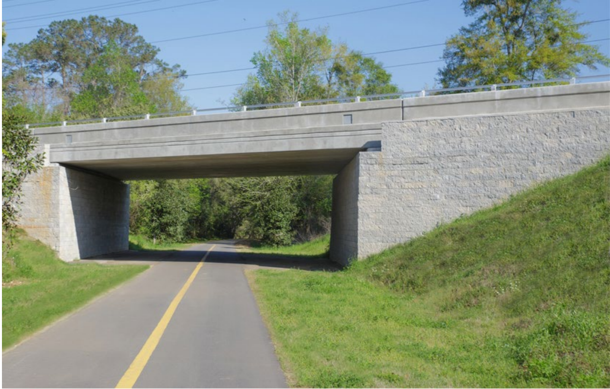
Figure 2-8. Orange Avenue Bridge in Tallahassee, Florida. ( https://ncma.org/updates/projects/florida-manages-orange-avenue-bridge-with-grs-ibs/ ).
