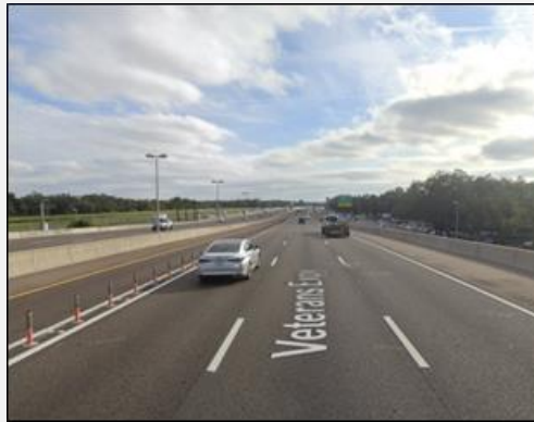
Veterans Exp: Pylons Separation
