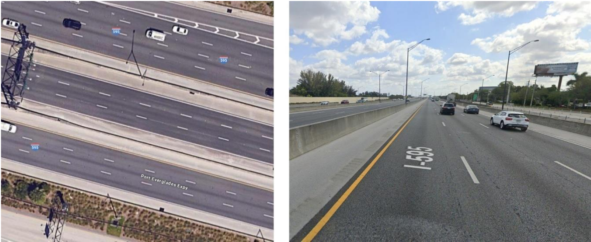
Figure 4.9: Site 7 – Concrete Barrier Separation (Three MLs) Link-Concrete(c)
