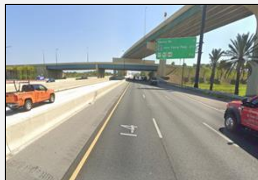
I-4: Concrete Barrier Separation
