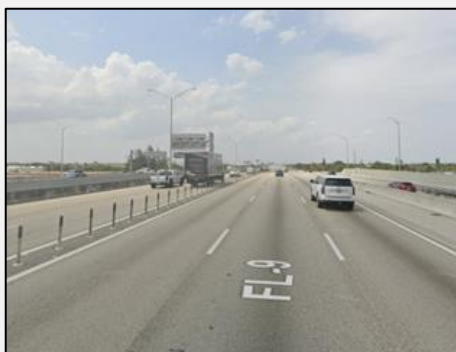
I-95: Pylons Separation
