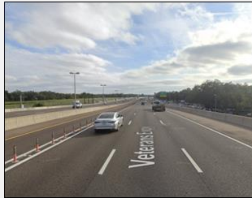
Veterans Exp: Pylons Separation
