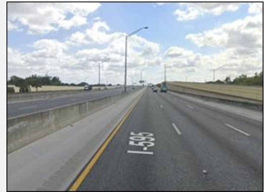
I-595: Concrete Barrier Separation
