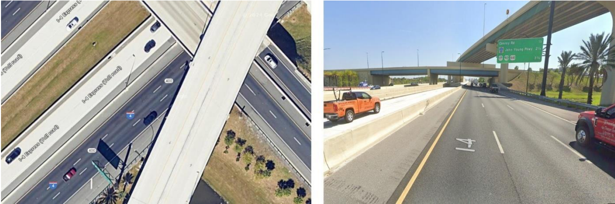
Figure 4.8: Site 6 – Concrete Barrier Separation (Two MLs) Link-Concrete(b)
