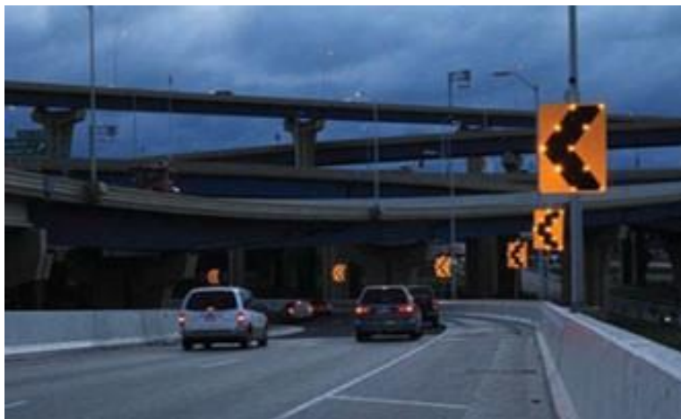
Figure 6.3: Sequential Dynamic Curve Warning Systems (SDCWS) (FHWA, 2016)
