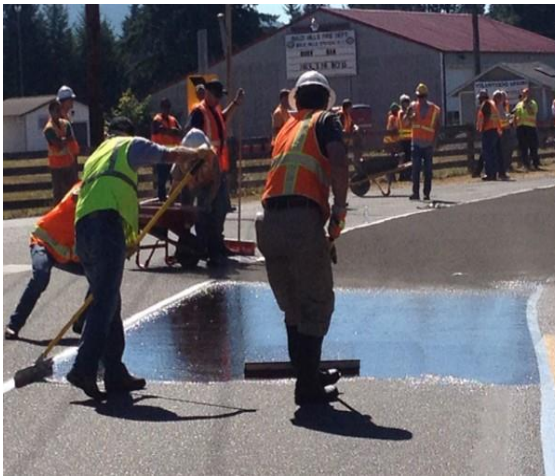
(a) HFST installation
