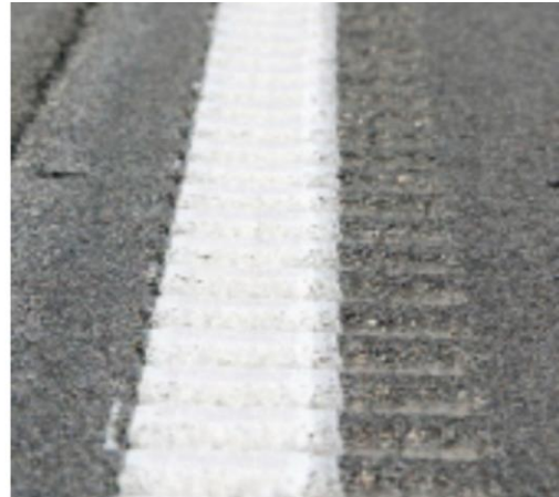
(b) Edge line rumble strips (FHWA, 2018)
