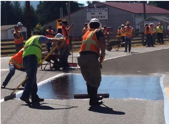
(a) HFST installation
