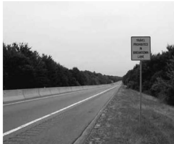
(b) Concrete median barriers Source: Gårder (2006)
