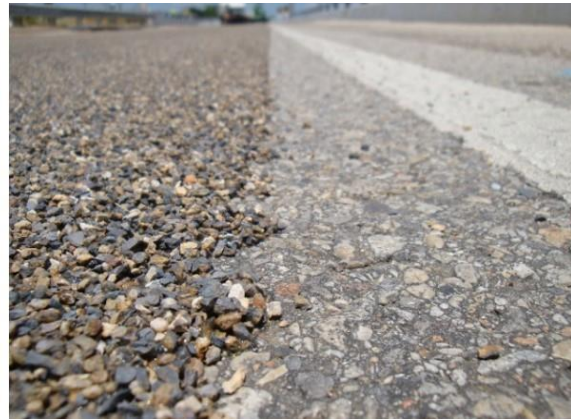
(b) HFST after installation
