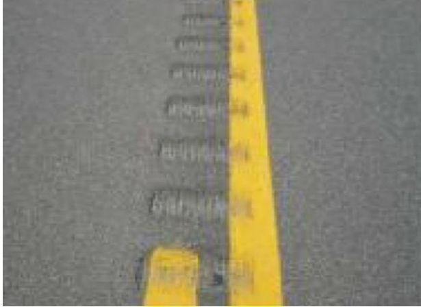
(a) Centerline rumble strips (FHWA, 2023)
