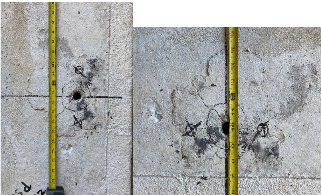
Figure A-8: P-SE1-2 specimen concrete after loading
