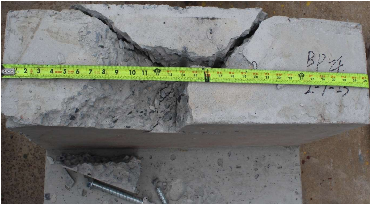
Figure A-103: B-P-4 specimen concrete after breakout
