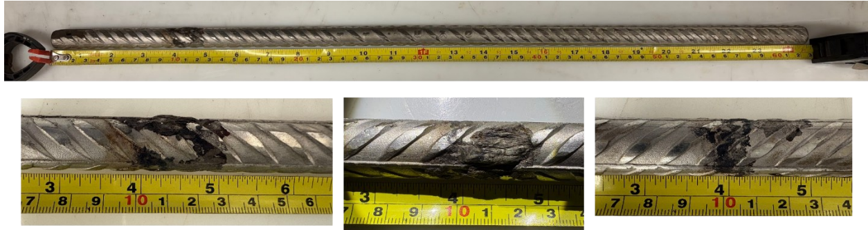
Figure 8-41. Full length of rebar 3 and notable areas of corrosion damage of sample STD3-2101-B.
