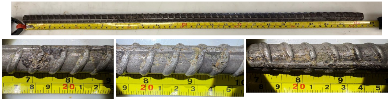
Figure 8-52. STD3-MMFX-B - full length of rebar 3 and notable areas of corrosion damage.
