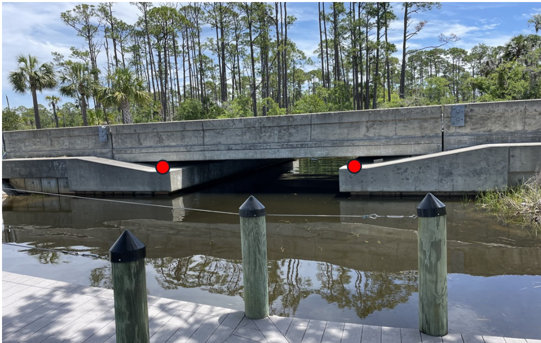
Figure 6-1. Picture of SR30A Bridge (510072) taken from the marina, left dot location 1, right dot is location 2.
