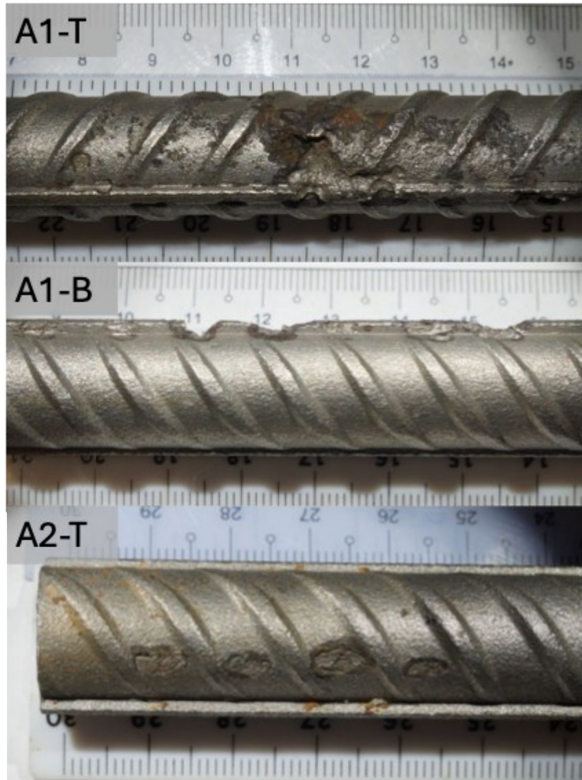
Figure 7-27. Rebars A1 and A2 closeups (top and bottom).
