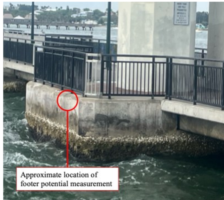
Figure 2-12. Approximate region where Jensen Beach Bridge footer potential measurements were taken.
