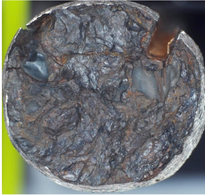
Figure 7-36. Corrosion of unclad, embedded rebar end of rebar C1 after cleaning.
