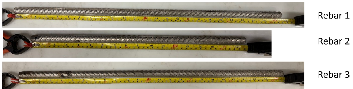
Figure 8-39. All rebars of sample STD3-2101-B after cleaning.
