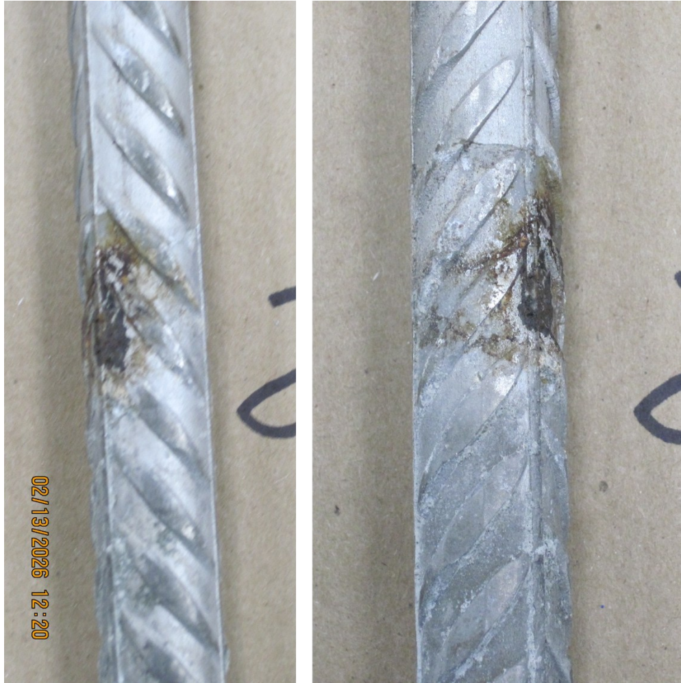
Figure 8-17. Close up of corrosion spot on rebar 2 of sample STD3-2101-B at multiple angles.
