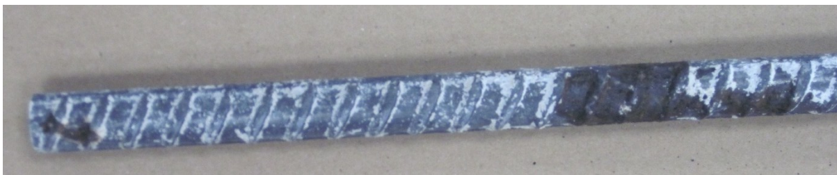
Figure 8-32. Corrosion spots observed on rebar 3 of sample STD3-MMFX-B.
