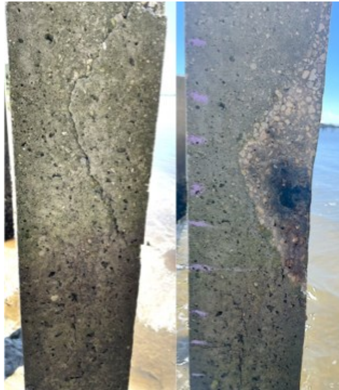
Figure 5-10. Picture showing north face of 2101-C in October 2024 (left) and September 2025 (right).
