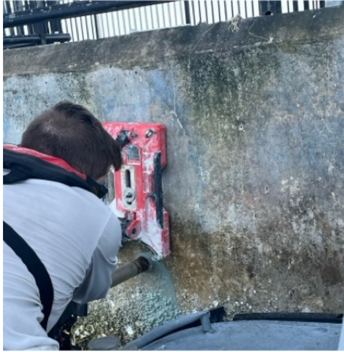
Figure 2-13. Coring of the north footer of Jensen Beach Bridge Pier 11, close to the marine growth.
