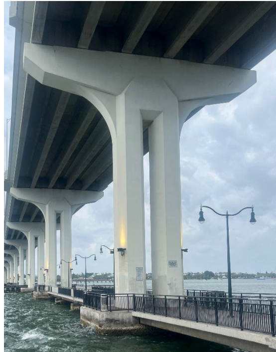
Figure 2-11. Photo of Jensen Beach Bridge Pier 12.
