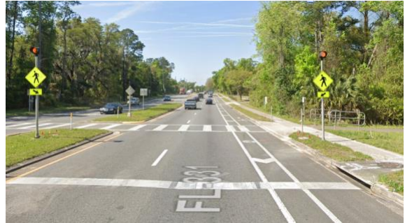
b. Flashing Beacon
