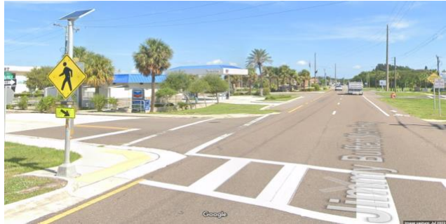
a. Rectangular Rapid Flashing Beacon (RRFB)
