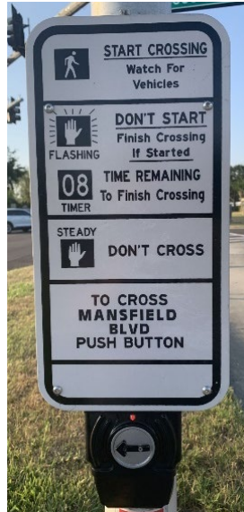
Figure 2-8. Example of pushbutton-integrated APS from various manufacturers
