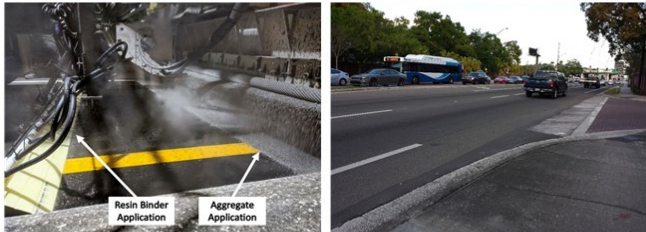
Figure 2-28. HFST construction and field photo at Hillsborough Ave @ N Central Ave, Tampa, Florida
