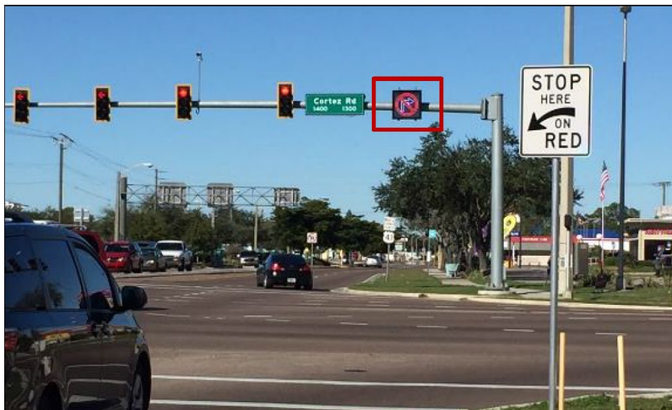
Figure 2-32. Site with "No Turn on Red" blank-out sign
