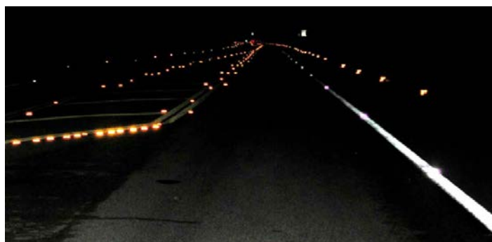
Figure 6-2 LEDs embedded in the road. (Image courtesy to: https://www.researchgate.net/figure/Embedded-roadway-lighting-These-LED-lights-installed-in-the-pavement-are-not-visible-to_fig24_305720851 )
