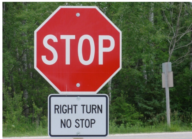
Figure 2-32 Stop sign with "Right Turn No Stop".
