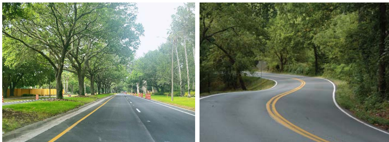
(a) Straight and clear lanes at daytime
