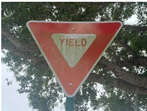
(a) Yield sign covered with dirt
