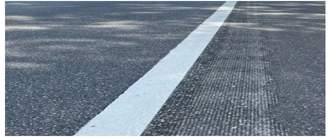
The research team selected Type 2 of three sinusoidal rumble strips designs as the most adequate for FDOT roadway departure needs, as seen here on a shoulder on SR-100.
