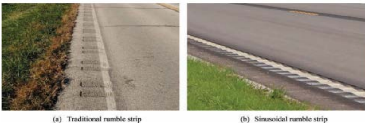
Figure 2-17. Traditional and sinusoidal rumble strip
