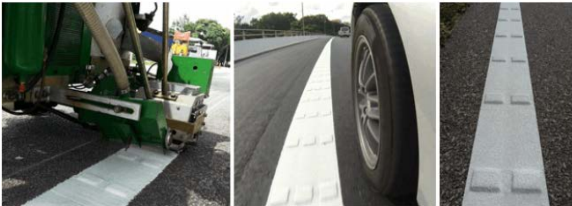
Figure 1-3. Examples of profiled thermoplastic rumble strips
