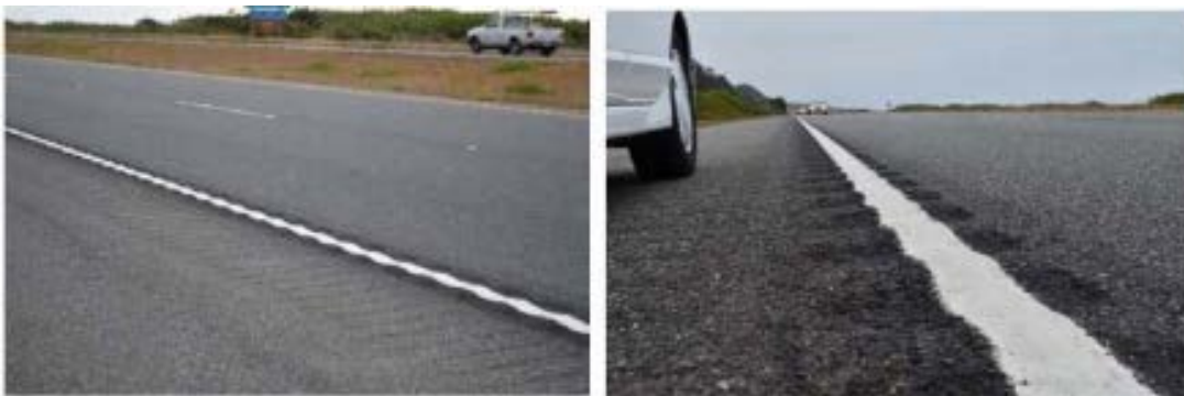
Figure 2-7. Mumble strips installed on US-101 (California)
