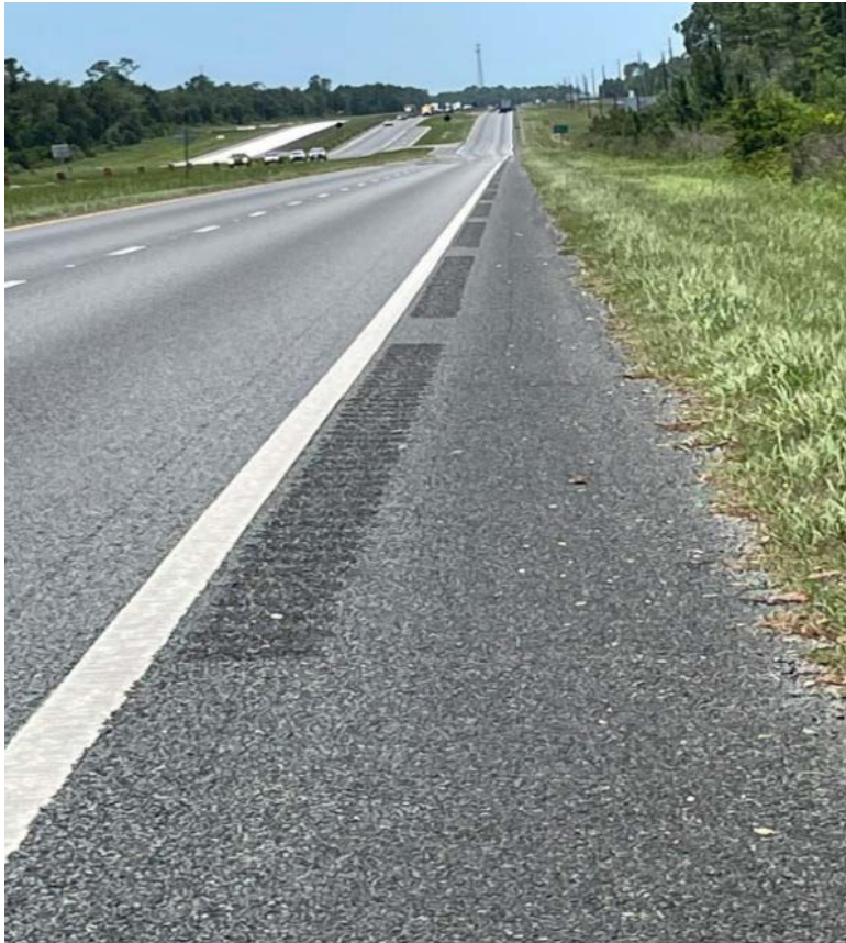
Figure 3-10. US-301 shoulder rumble strip Type 1
