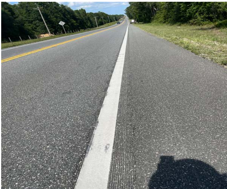
Figure 3-16. SR-100 edgeline rumble strip Type 2
