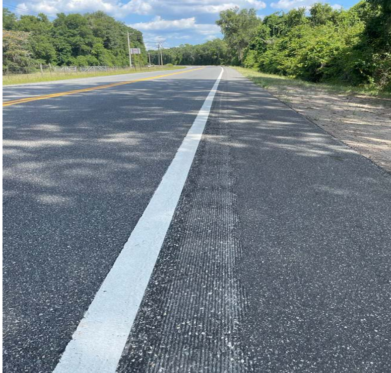
Figure 3-13. SR-100 shoulder rumble strip Type 2
