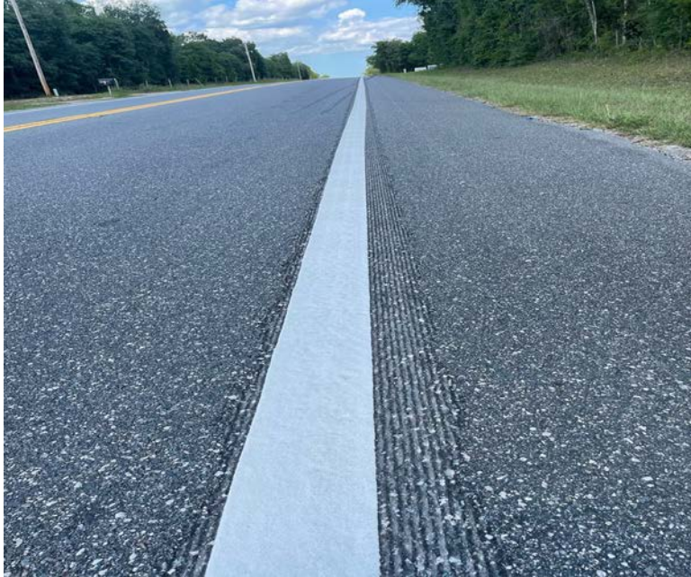
Figure 3-15. SR-100 edgeline rumble strip Type 1
