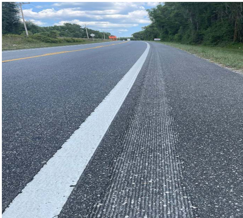
Figure 3-12. SR-100 shoulder rumble strip Type 1
