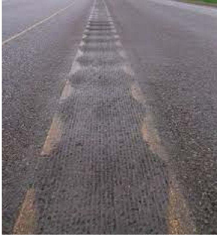
Figure 1-6. Example of sinusoidal rumble strip
