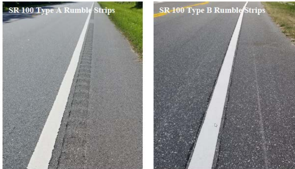
Figure 3-24. Comparison of SR-100 rumble strips between Type A and Type B
