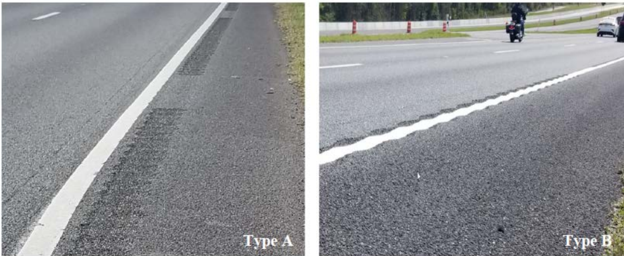
Figure 3-20. Comparison of US-301 rumble strips between Type A and Type B
