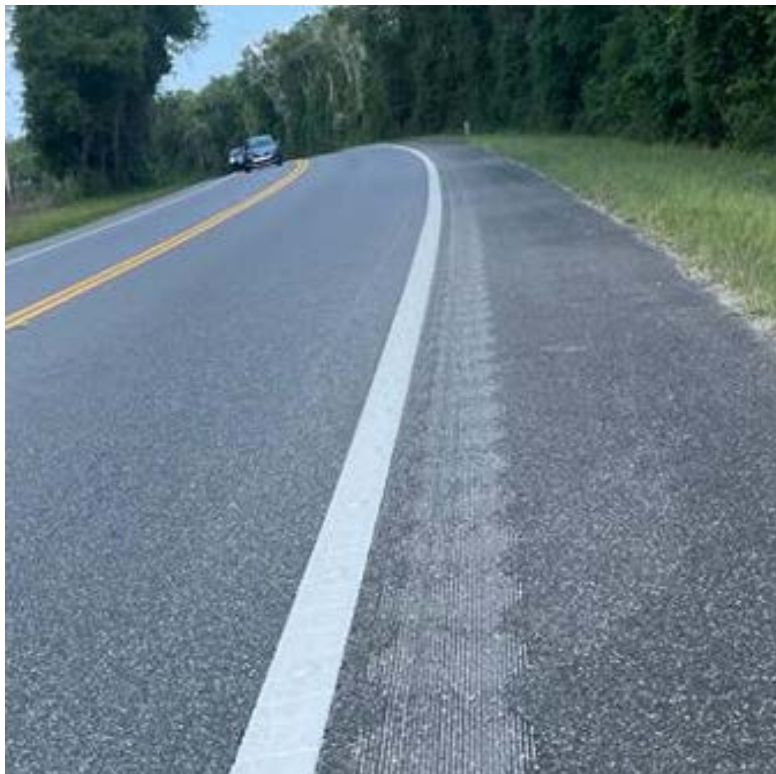
Figure 3-14. SR-100 shoulder rumble strip Type 3
