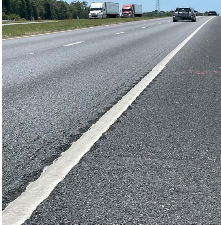
Figure 3-11. US-301 edgeline rumble strip Type 3
