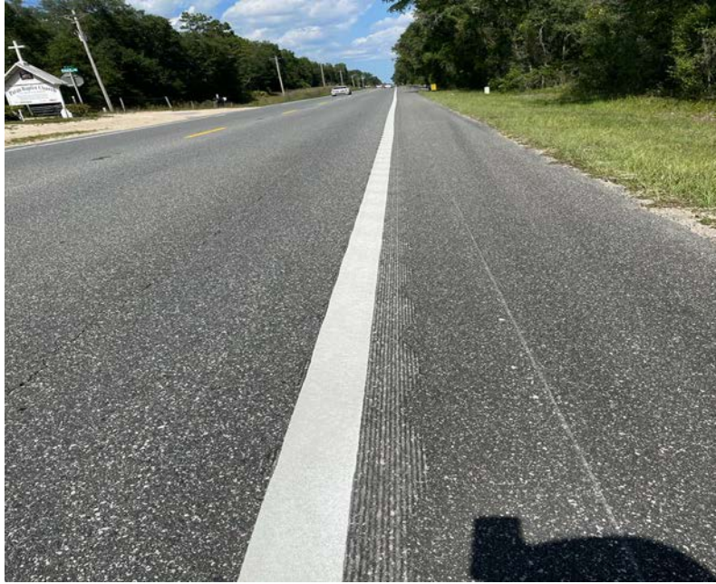
Figure 3-17. SR-100 edgeline rumble strip Type 3
