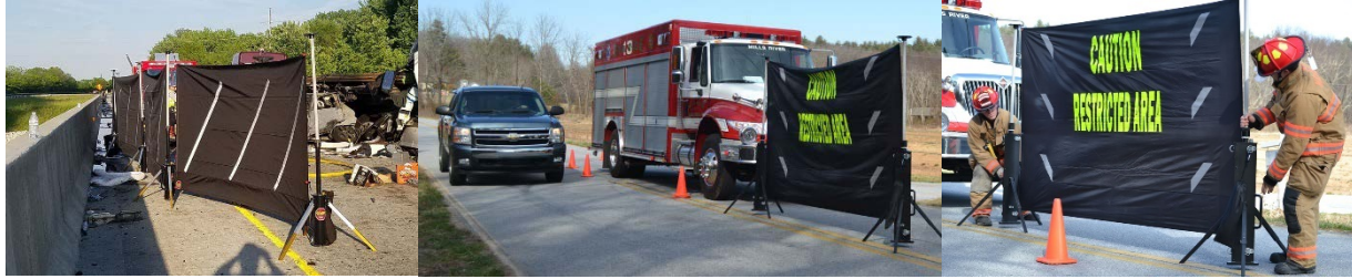
Figure 2-9. GawkStopper deployment examples
