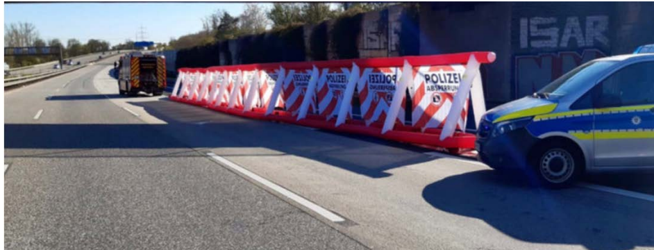
Figure 2-11. Privacy screen used in Germany
