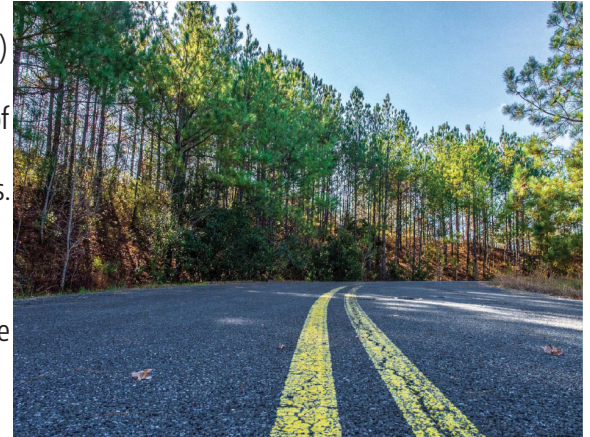
FDOT uses an open-graded friction course known as FC-5. The research from BEB15 provides an assessment of strategies designed to improve the durability of FC-5 mixtures.
