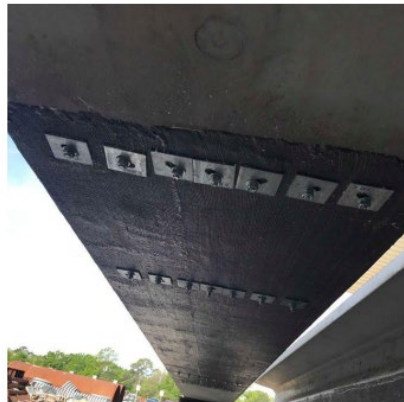
Figure 27: Mechanical plate anchors for girder (Aljaafreh, Performance of Precast Concrete Bridge Girders with Externally Bonded Anchored CFRP, 2019)
