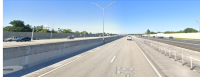
Concurrent Flow Express Lanes along I-75 in Florida.
