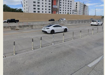
Managed lanes with pylons separation
