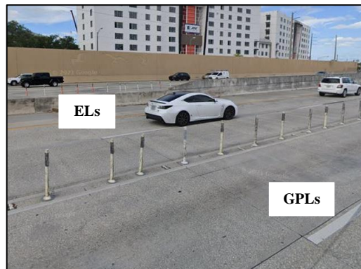
(b) Pylons on I-95
