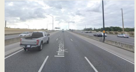
Managed lanes with concrete barrier separation
