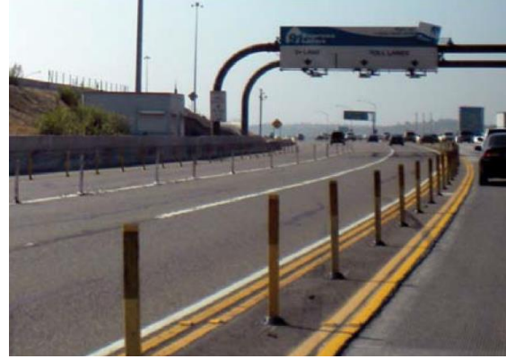
(b) Individual Pylon Separation on the SR-91 Express Lanes
