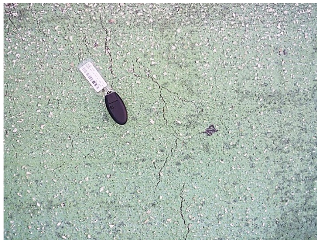
Figure 3-3. Worn-Out MMA.
