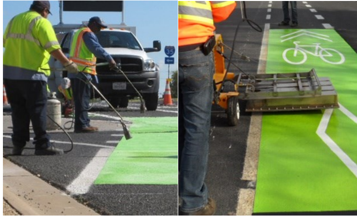
Figure 2-10. Installation Methods of Preformed Thermoplastic. (NACTO, 2020)
