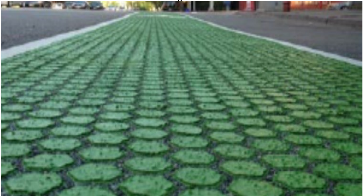
Figure 2-5. Polymer Cement Slurry. (Tensar International, 2021)
