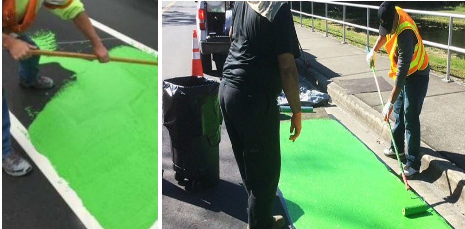
Figure 2-13. Installation of MMA. (Anderson et al., 2018; Transpo Industry)
