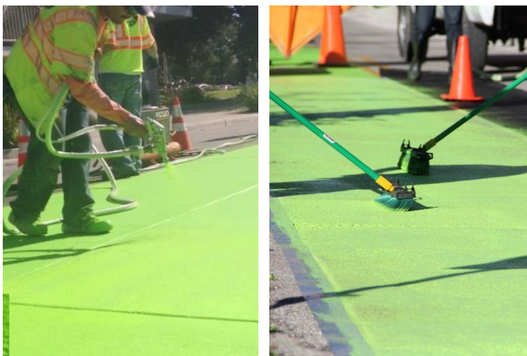
Figure 2-11. Manual Spray and Brush Application of Epoxy-Modified Acrylic.
