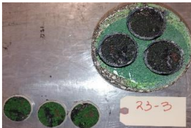
Figure 3-10. Clean Delamination under Pull-Off Test.
