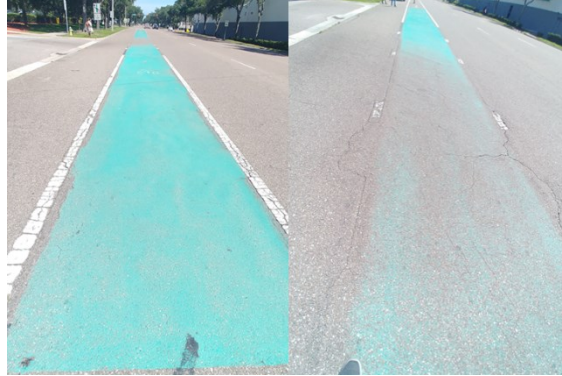
Figure 2-4. Paint Treated Bike Lane in Pittsburg, Florida.
