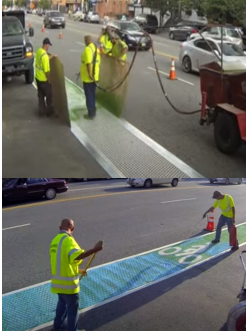
Figure 2-15. Installation of Polymer Cement Slurry. (Tensar International, 2021)
