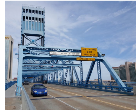
Jacksonville's Alsop Bridge is one of hundreds of steel bridges in Florida that require regular painting, requiring hundreds of work hours and thousands of gallons of paint.
