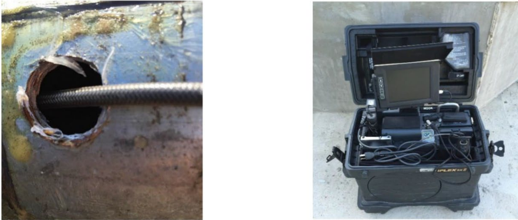
Figure 46. Borescope access port and equipment used (Hurlebaus et al. 15 )
