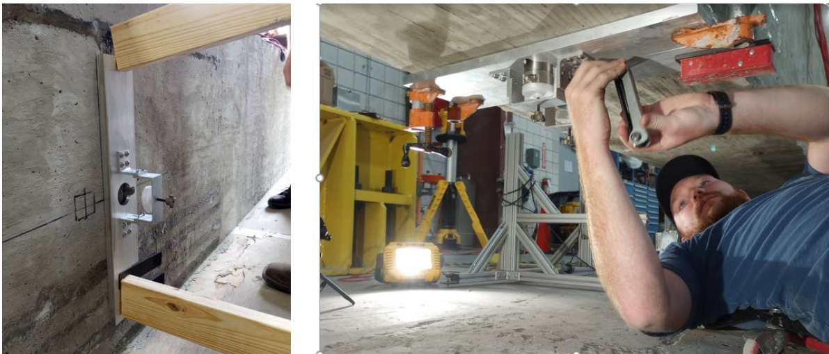
Figure 134. Fixture for mounting transducers using two-part epoxy
