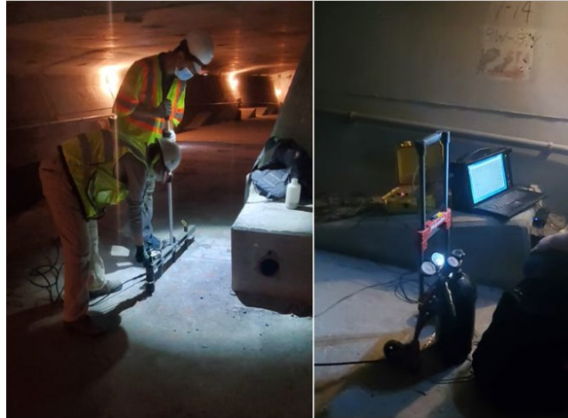
Figure 7. Impact echo testing across closure pour. Seabreeze Bridge, Daytona Beach
