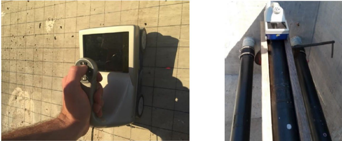
Figure 29. StructureScan Mini HR GPR unit inspecting concrete and the external tendons (Hurlebaus et al. 15 )
