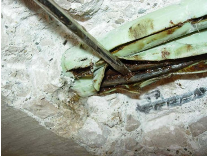
Figure 59. Exposed tendon after strand rupture in office-building roof (Shear et al. 48 )
