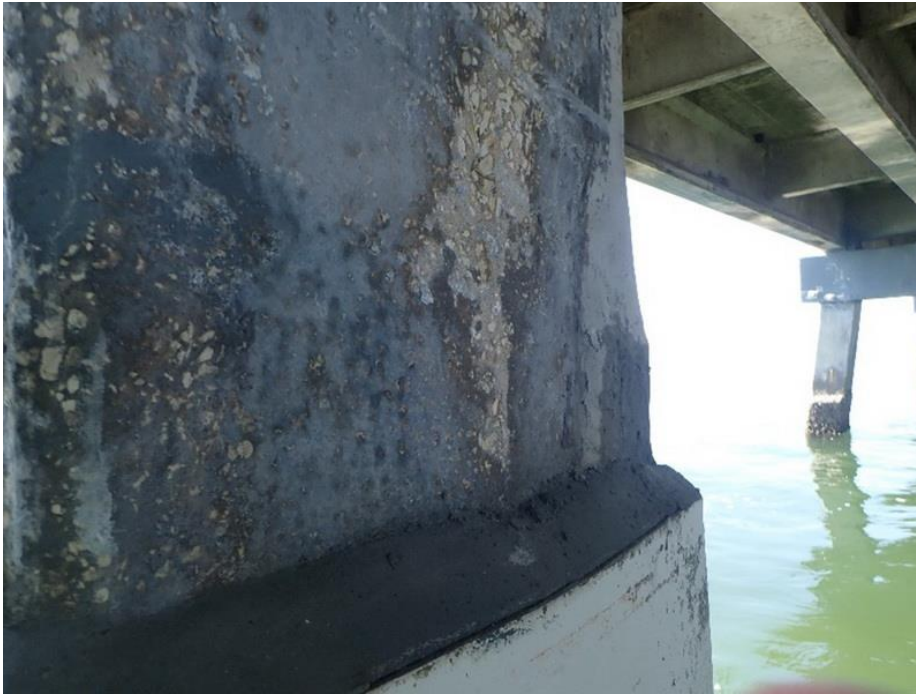
Figure 87. Repair on NW corner of the pile (Pile 138-7)
