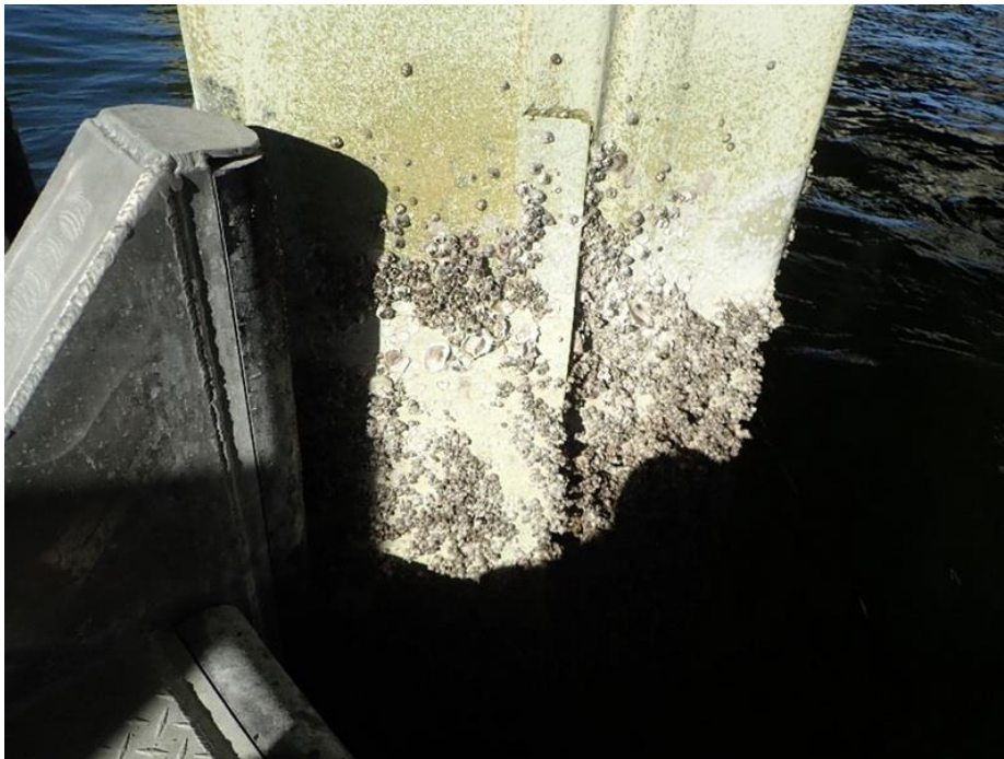
Figure 106. Jacket opening at the bottom (Pile 85-4)
