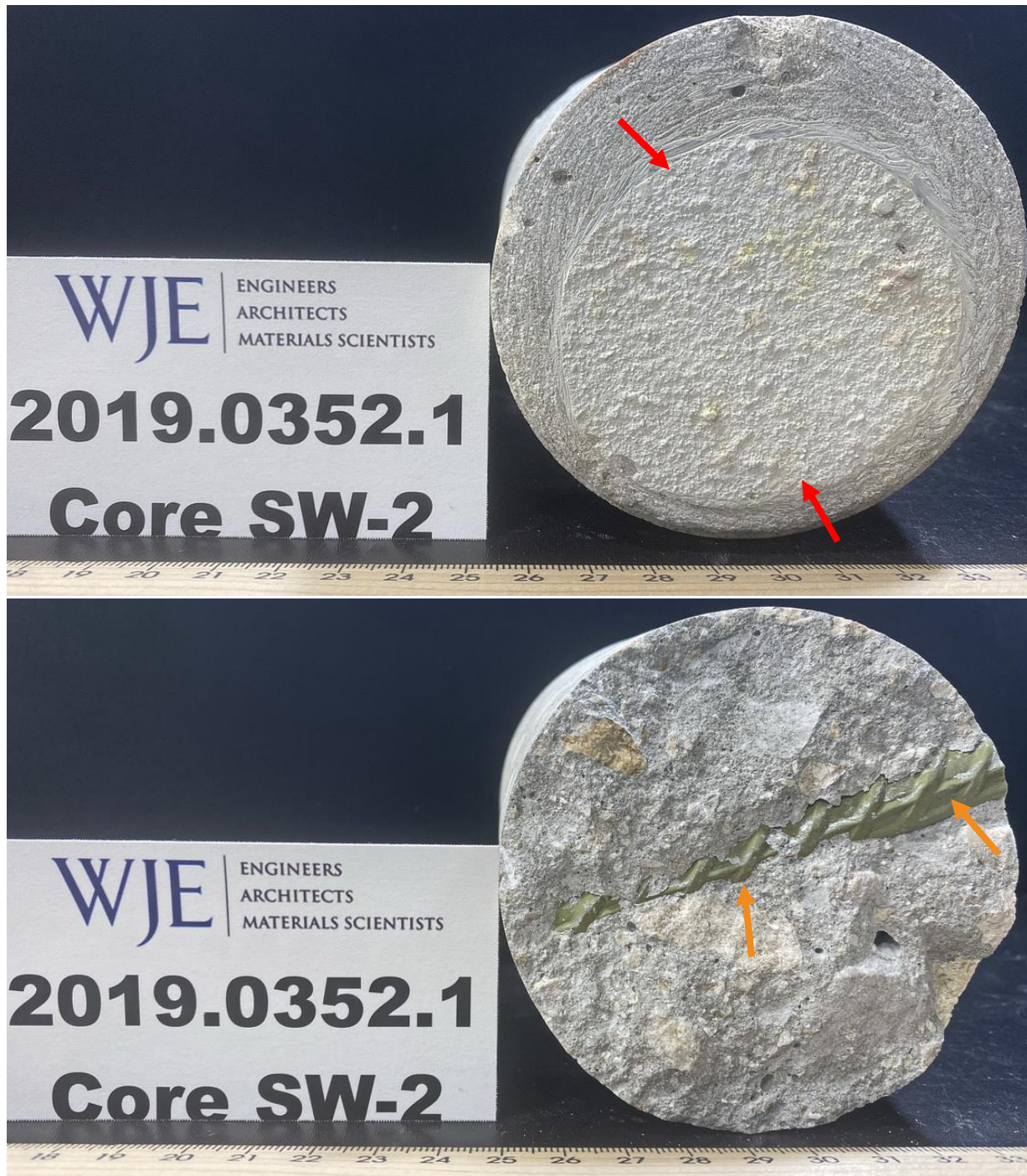
Figure 127. Core SW-2. Exterior (exposed) surface (top photo) and interior surface (bottom). The interior fractured surface extended mainly through coarse aggregate particles, consistent with a tight paste-aggregate bond. Orange arrows indicate a partially exposed No. 5 reinforcing steel bar.
