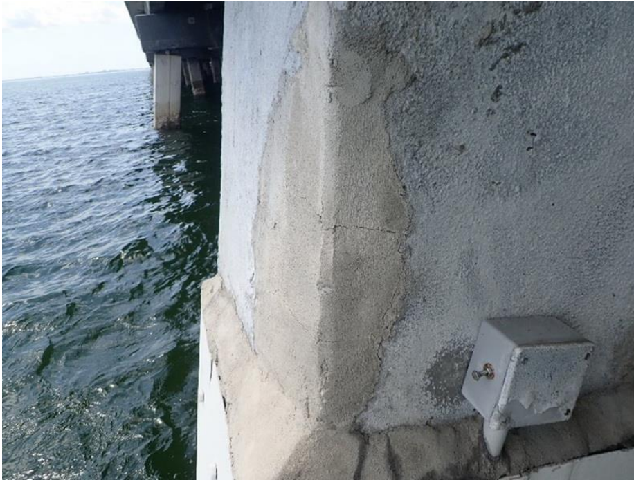
Figure 103. Repair on pile corner (Pile 316-8)
