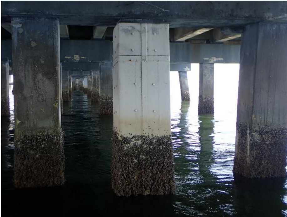
Figure 85. Jacket extension on top, no distress noted (Pile 129-6)
