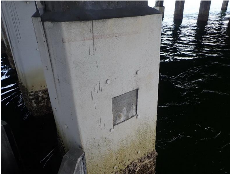
Figure 99. Overview photograph of pile and jacket with no noted distress (Pile 289-2)
