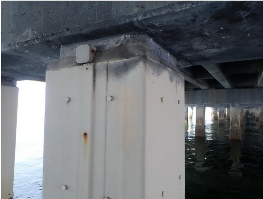
Figure 81. Overview photograph of pile and jacket with no noted distress (Pile 116-4)
