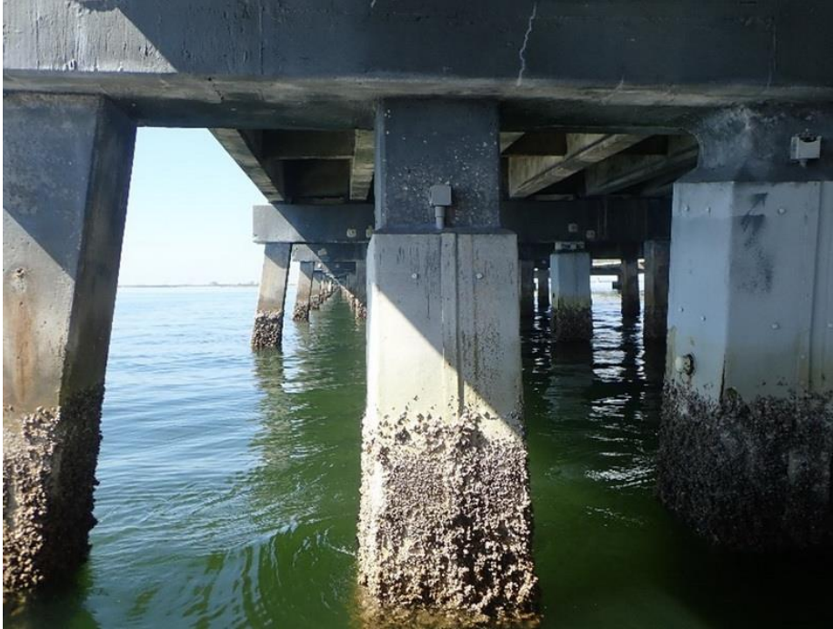
Figure 79. Overview photograph of pile and jacket with no noted distress (Pile 99-9)
