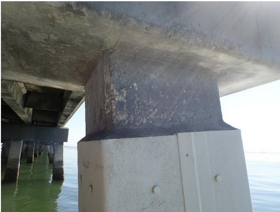
Figure 76. Overview photograph of pile and jacket with no noted distress (Pile 65-8)
