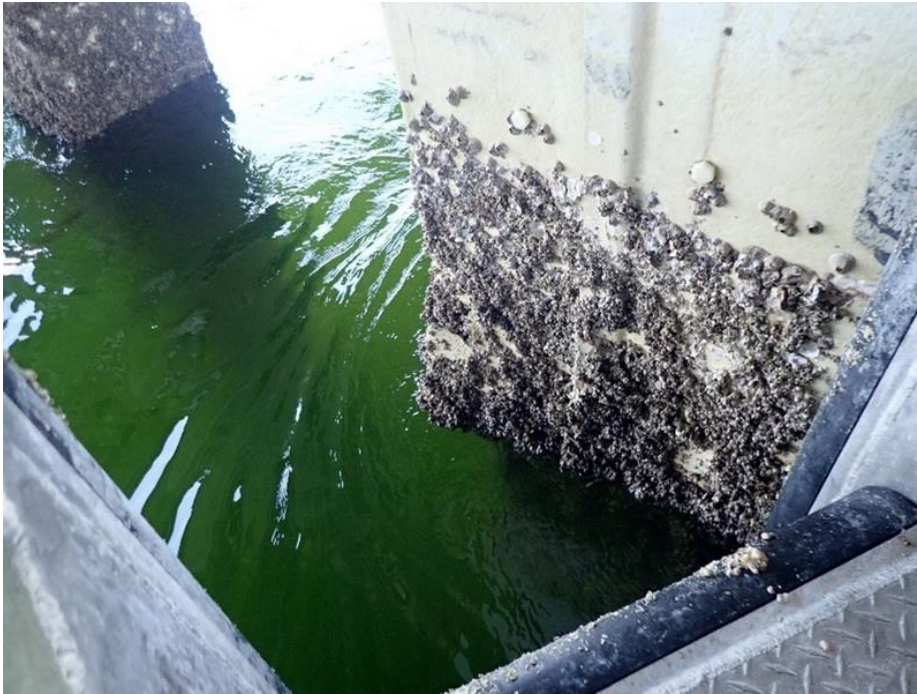
Figure 89. Horizontal splitting of jacket (Pile 177-4)
