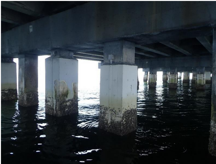
Figure 94. Overview photograph of pile and jacket with no noted distress (Pile 214-3)
