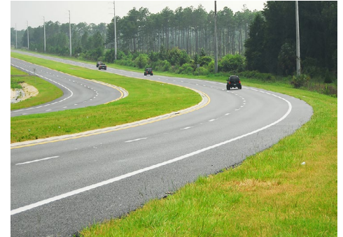
The ribbons of asphalt roadway that connect virtually all points in Florida are designed to last many years with a minimum of maintenance.
