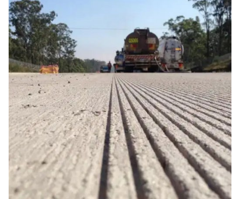
Tining, or adding groves to concrete pavement, improves traction but makes measuring macrotexture difficult.
